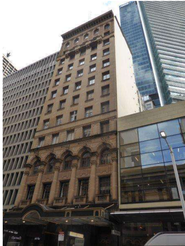
Figure 3 Castlereagh Street façade.
