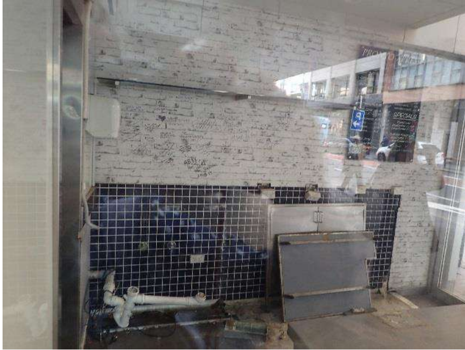
Figure 6 View into vacant shop at street level. Option 3 is to locate the monitoring equipment to attach to the wall abutting with the Masonic Club.
