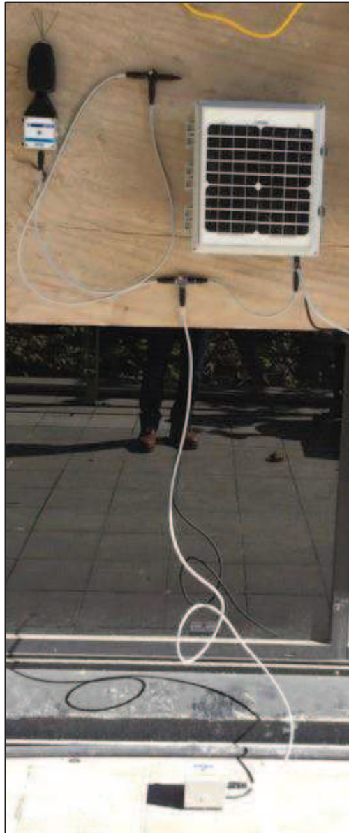
Figure 2 Typical layout of the vibration monitoring equipment.
