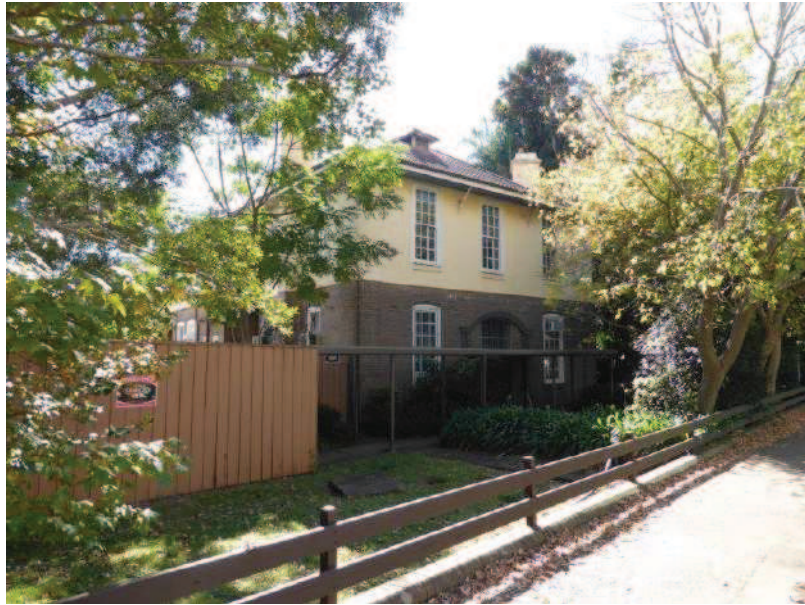
Figure 3 View north-east to Mowbray House.
