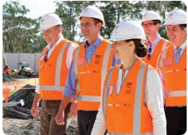
Premier Mike Baird, Minister for Transport Gladys Berejiklian and North West Sydney MPs inspect Cherrybrook tunnelling site in April 2014.
