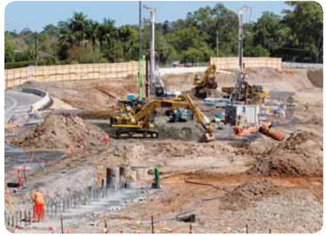
Excavation at the Cherrybrook construction site.
