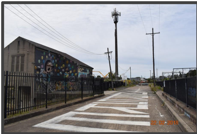
Image 2: Image taken from Railway Parade (South Eastern side of the site) looking towards the Drainage station and telecommunications facility.
