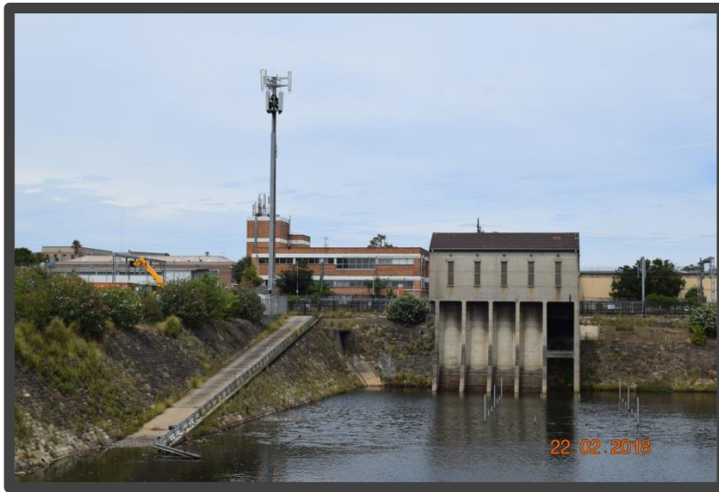
Image 1: Looking directly across the Sydenham Pit & Drainage Pumping Station from the North North-Western boundary
