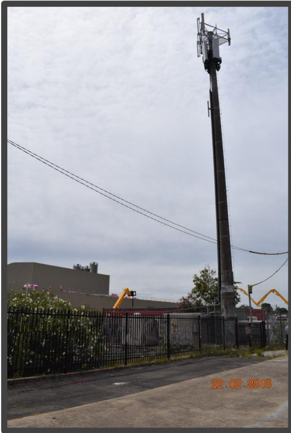
Image 3: Image of the telecommunications facility from Railway Parade facing north.
