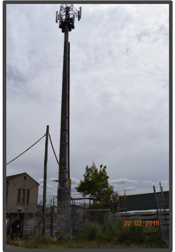
Image 4: Image of the telecommunications facility from Railway Parade facing west.
