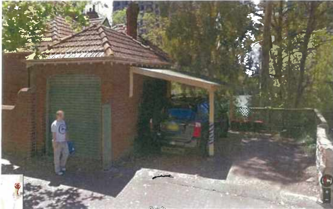
Figure 3. Garage and carport. Source TfNSW/Google Streetview
