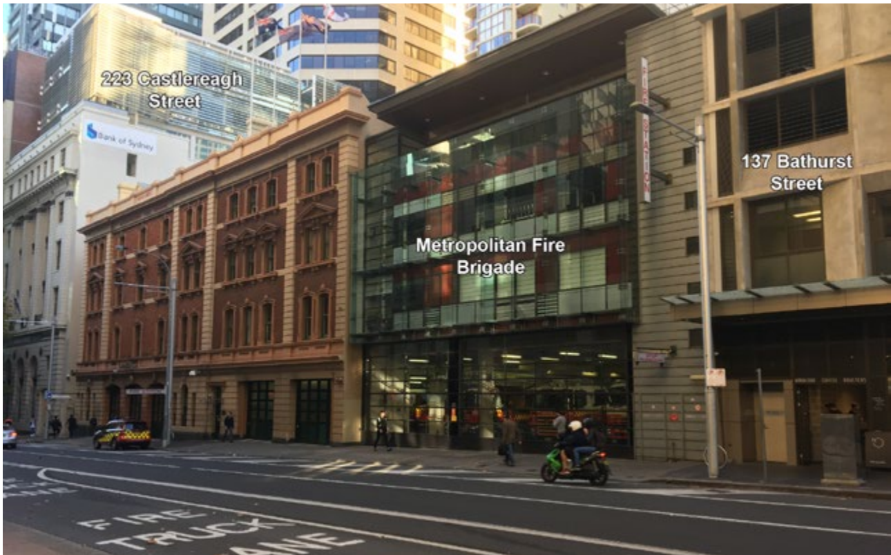
Figure 26 – Existing Metropolitan Fire Brigade building to the east of the site, as viewed from Castlereagh Street
