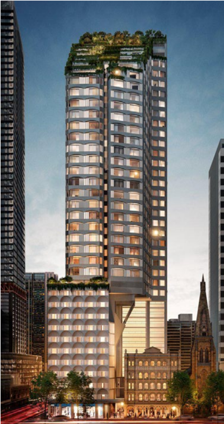
Figure 23 – ‘Castle Residences’, located at 110-118 Bathurst Street and under construction
