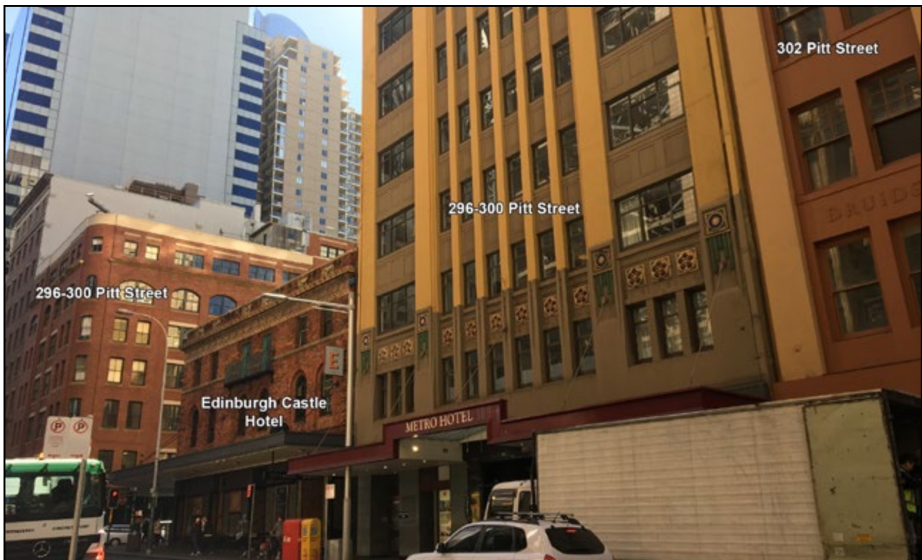
Figure 18 – Former development of the site, as viewed from Pitt Street (to the south)
