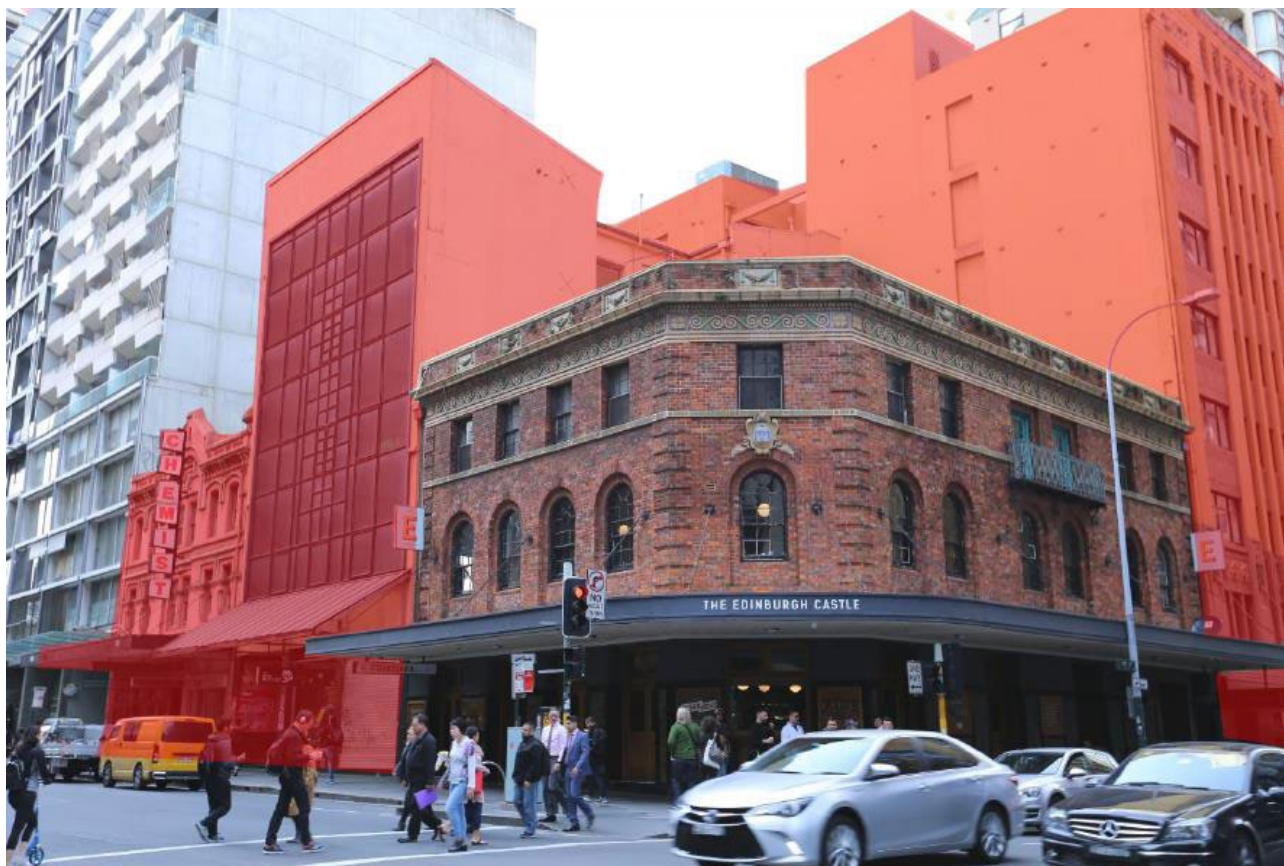
Figure 76 – View of the site (shaded in red), facing south-east, showing existing buildings and adjoining Edinburgh Castle Hotel at the corner of Pitt Street and Bathurst Street
