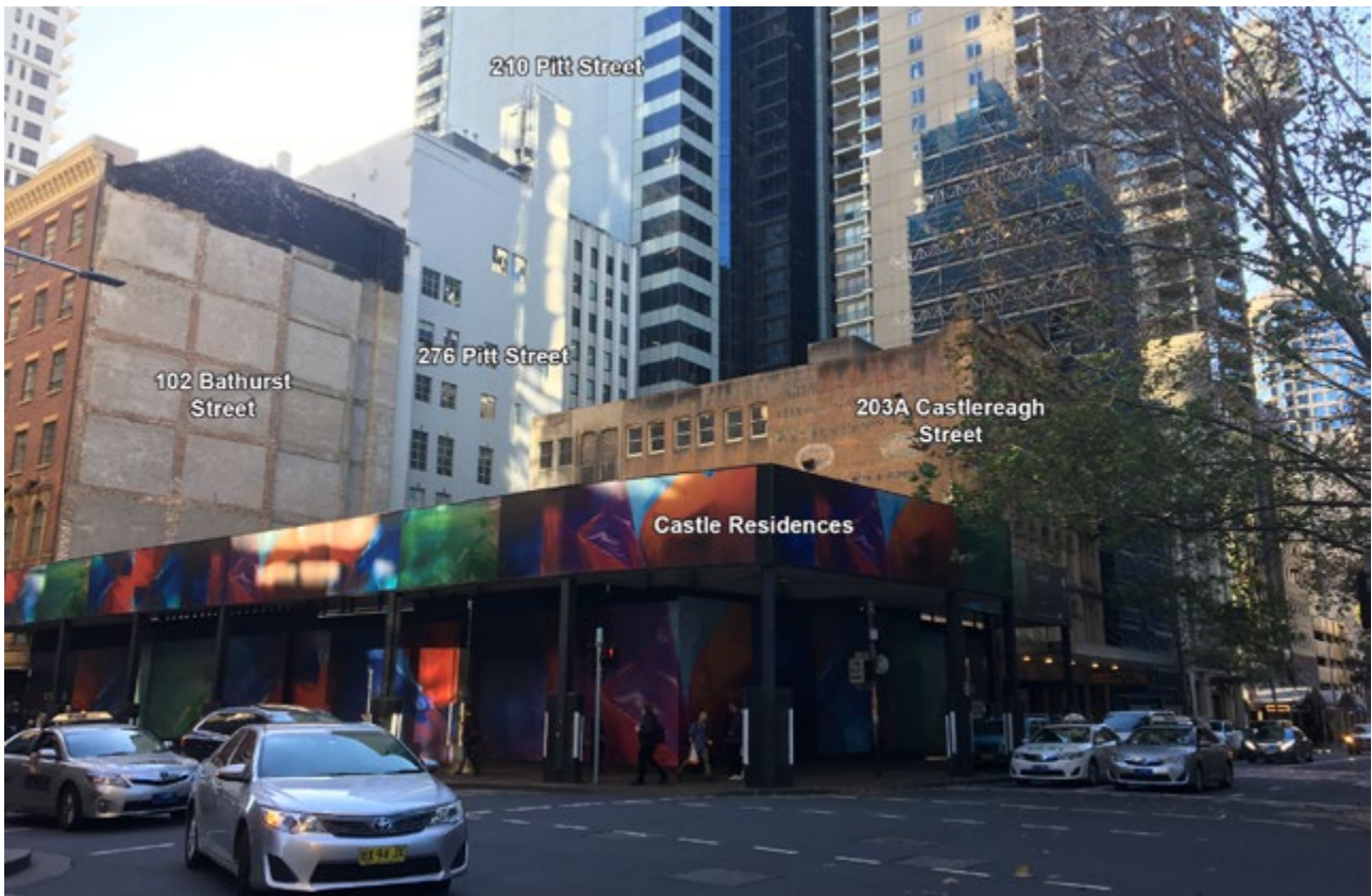
Figure 22 – The existing development along the northern side of Bathurst Street
