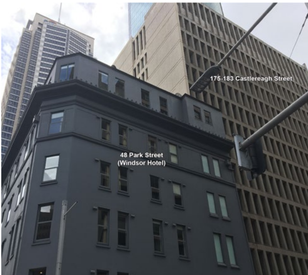
Figure 23 – Former development at the site, as viewed from the intersection of Park Street and Castlereagh Street
