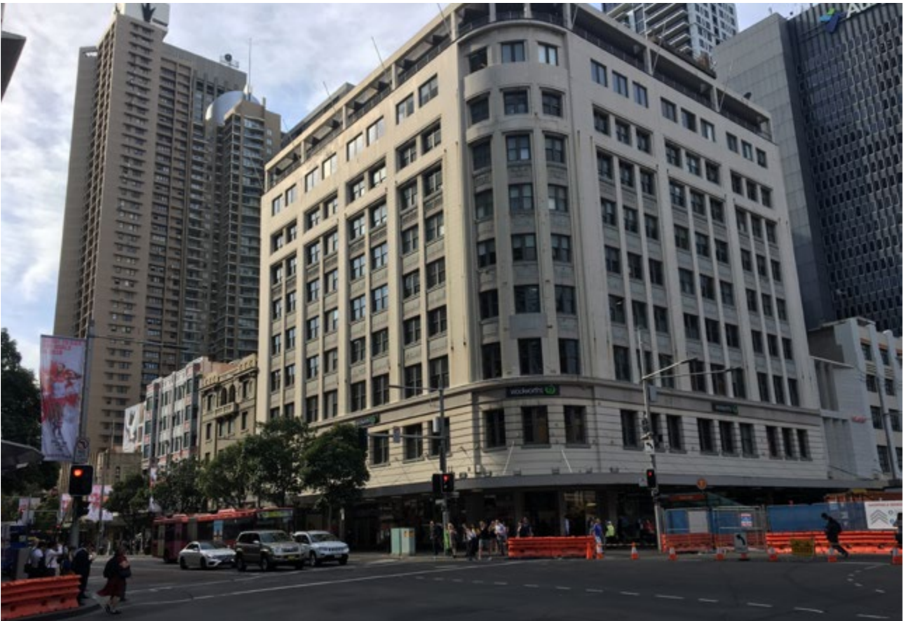
Figure 29 – Existing buildings at the site of the future Town Hall Square, to the south-west of the site (as viewed from George Street)
