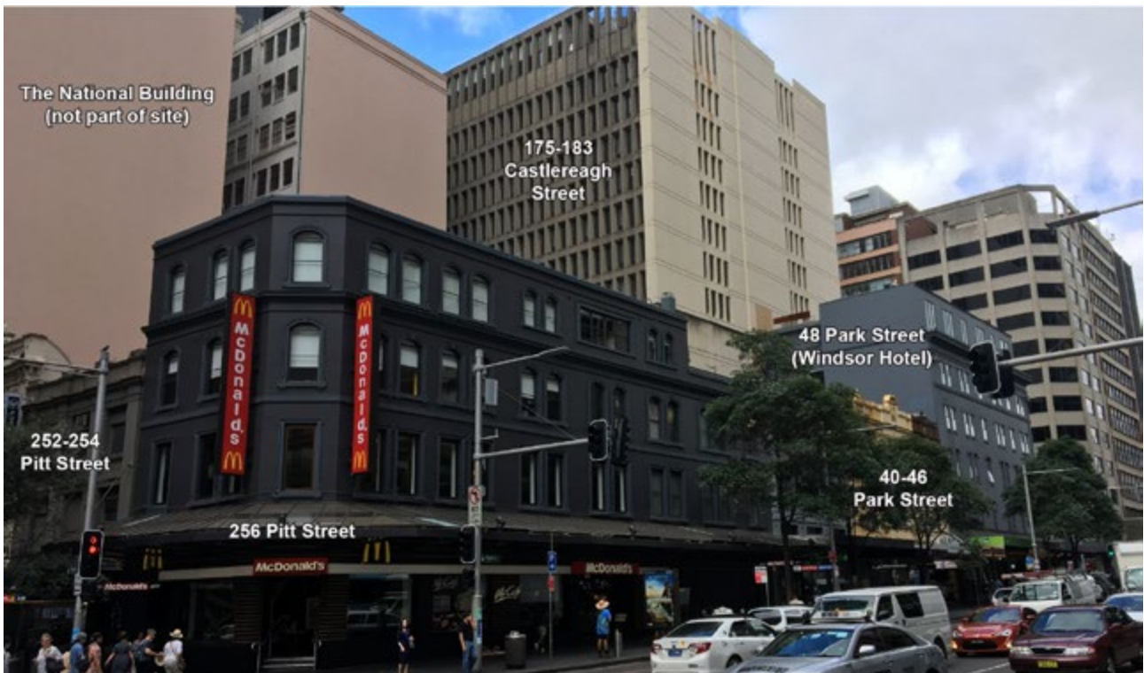
Figure 22 – Former development at the site, as viewed from the intersection of Park Street and Pitt Street
