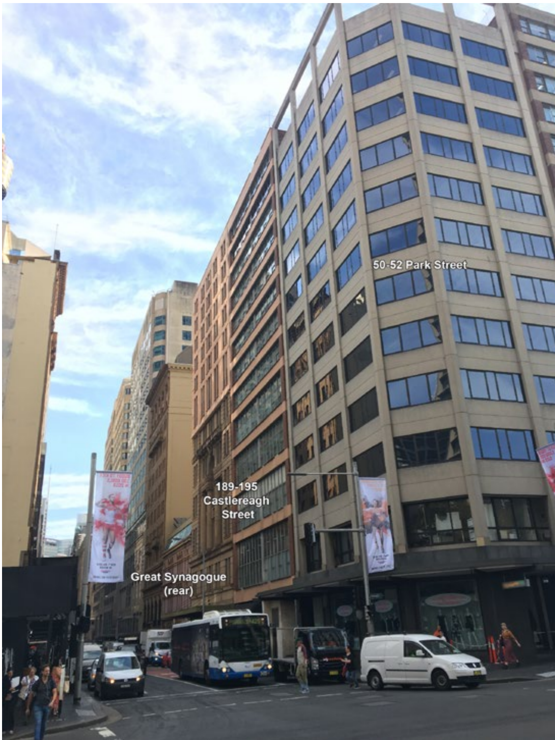
Figure 27 – Existing development to the east of the site, and Castlereagh Street
