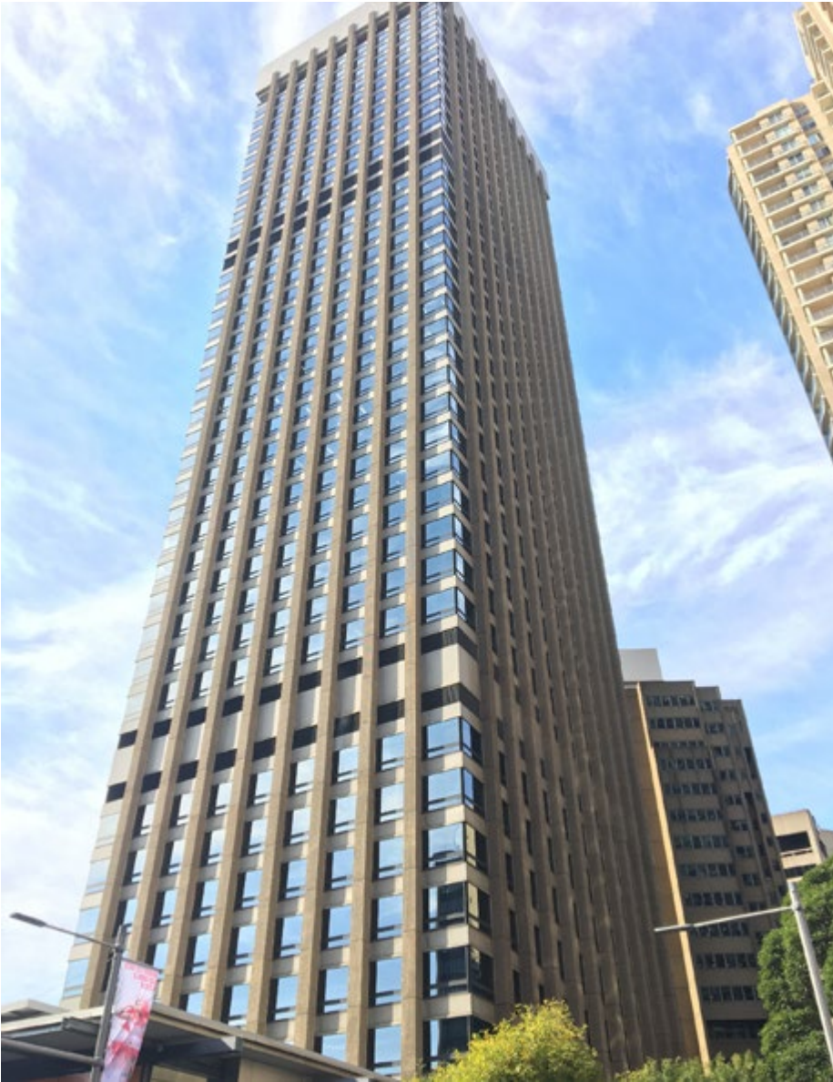
Figure 28 – Existing development at 201 Elizabeth Street
