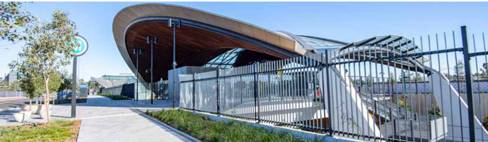
Bella Vista Station.
