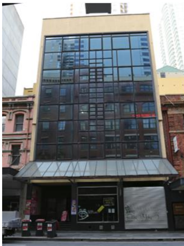
Figure 35 – The existing building after its mid-twentieth-century remodel
