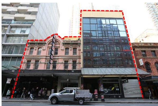
Figure 3 – View of two adjoining buildings along the southern alignment of Bathurst Street, which form part of the subject site Source: Urbis
