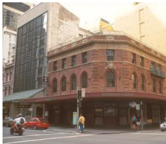
Figure 37 – Photograph of the subject site with the adjoining Edinburgh Castle Hotel in the centre, dated 19 March 2000
