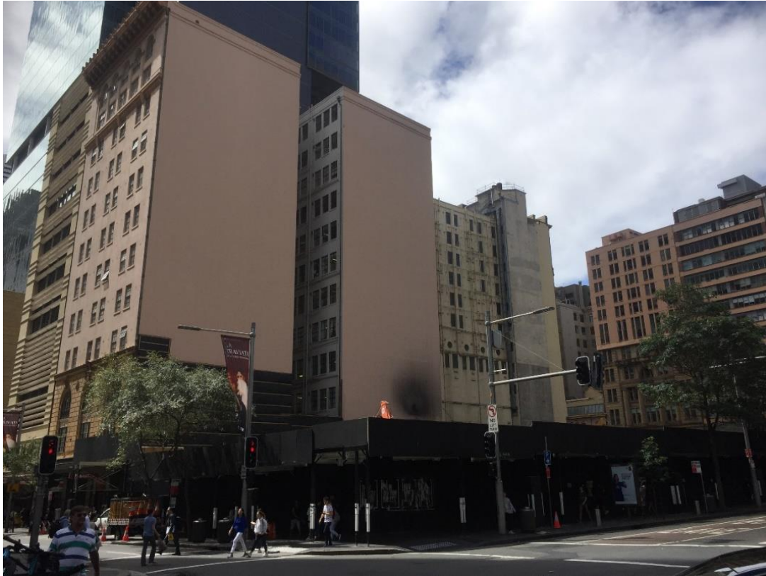
Figure 10: View of over station site from southwest with National Building at left and former Masonic Club at right. This photograph was taken after the State Significant Infrastructure demolition of buildings on the site.
