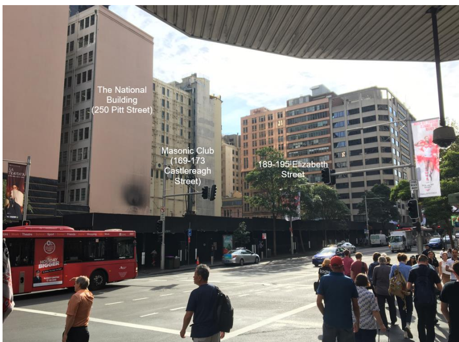
Figure 10: Existing development of the site, as viewed from Park Street (to the north east)
