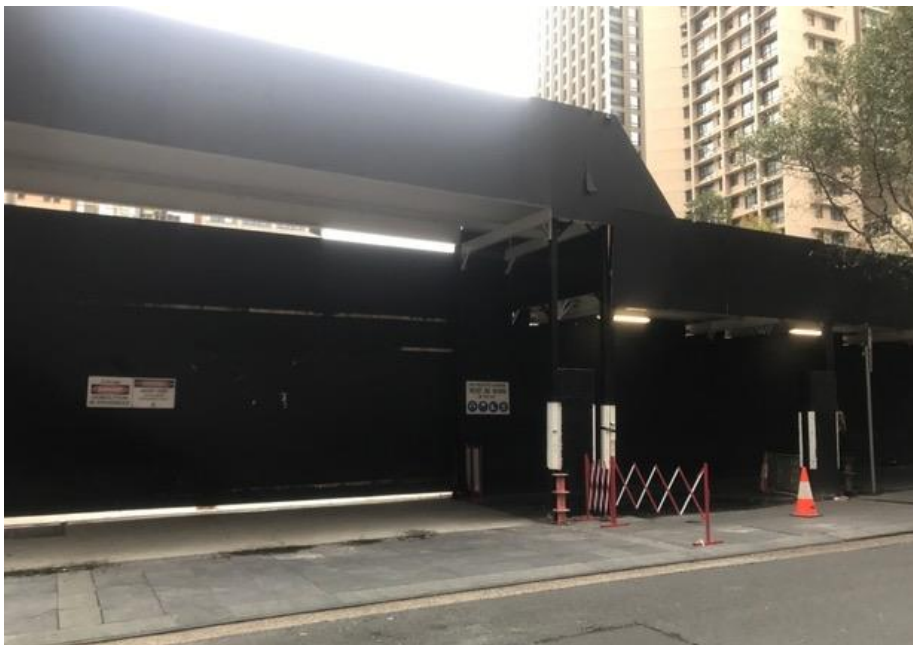
Figure 5: Existing site viewed from the secondary frontage of Pitt Street
