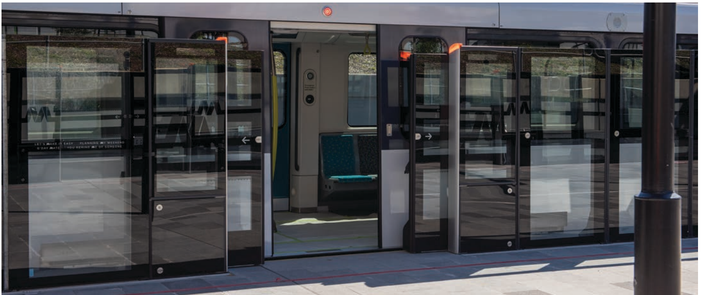
Australian first – platform screen doors
