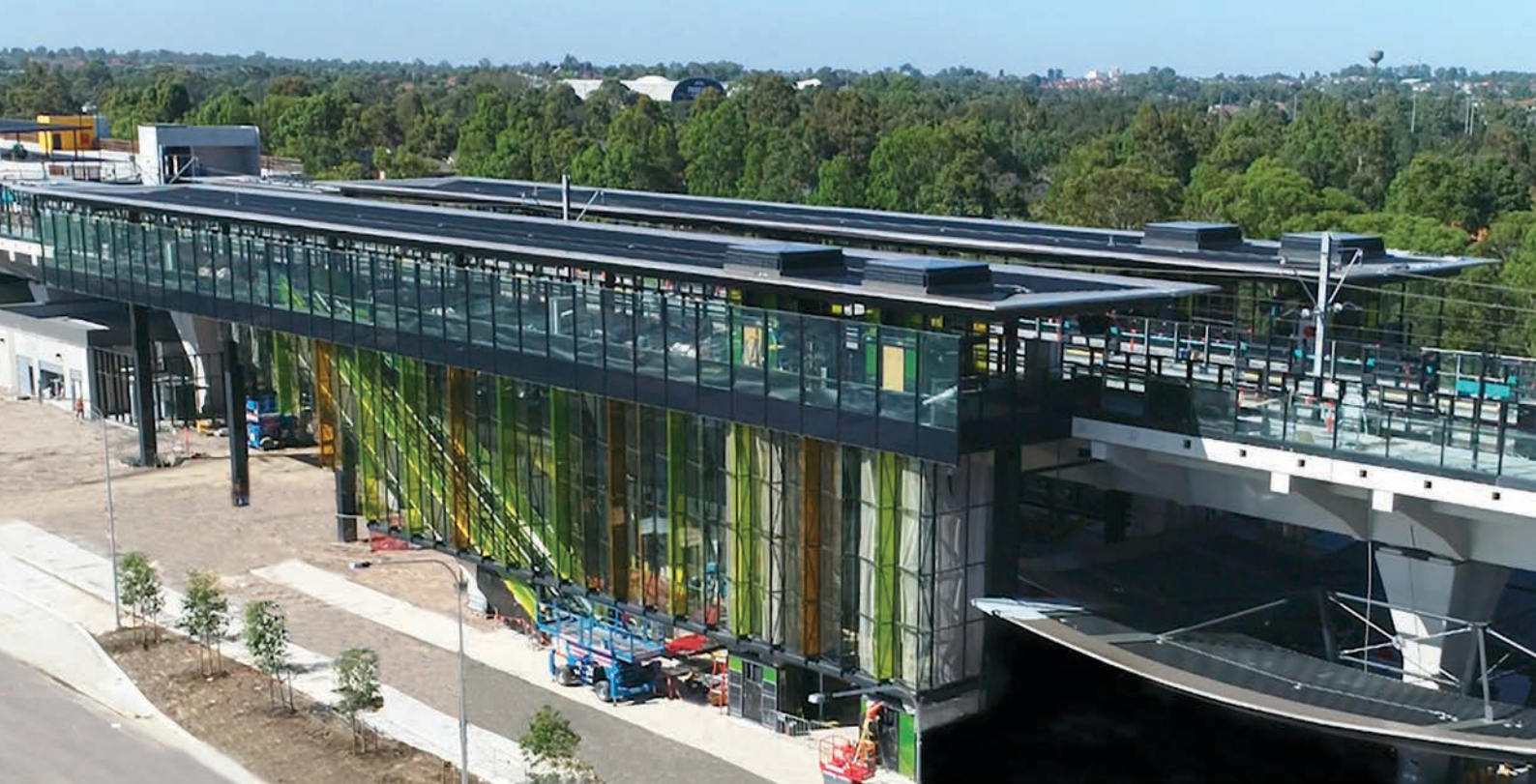
The new Kellyville Station and its iconic wall of glass
