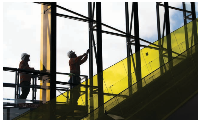
Workers installing glass at Kellyville Station
