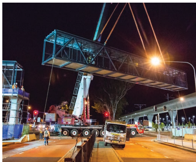
Bridge lifted into place over Windsor Road at Kellyville
