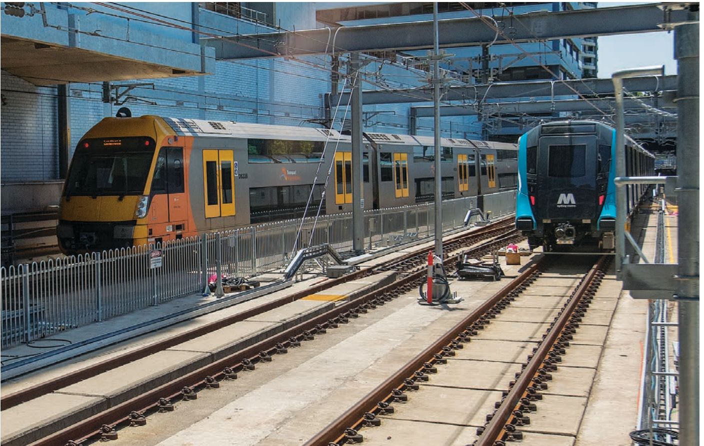
The first metro train (right) at Chatswood Station, alongside a suburban Sydney train
