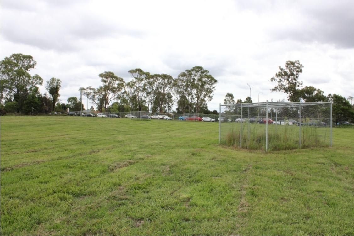
Photograph 3.1 Kellyville Station construction area looking towards Windsor Road. Two of the well locations are visible in this photograph.
