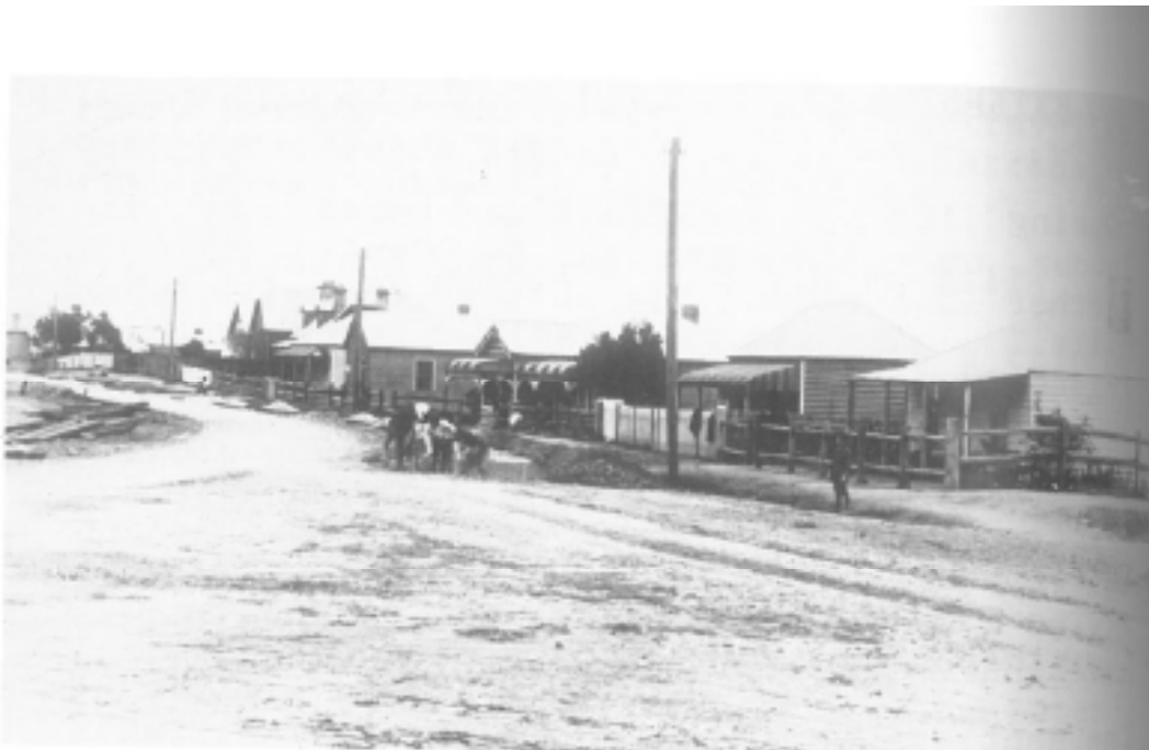
Photograph 2.2 Laying of the tram tracks in 1909 (source: Hills District Historical Society 1990)
