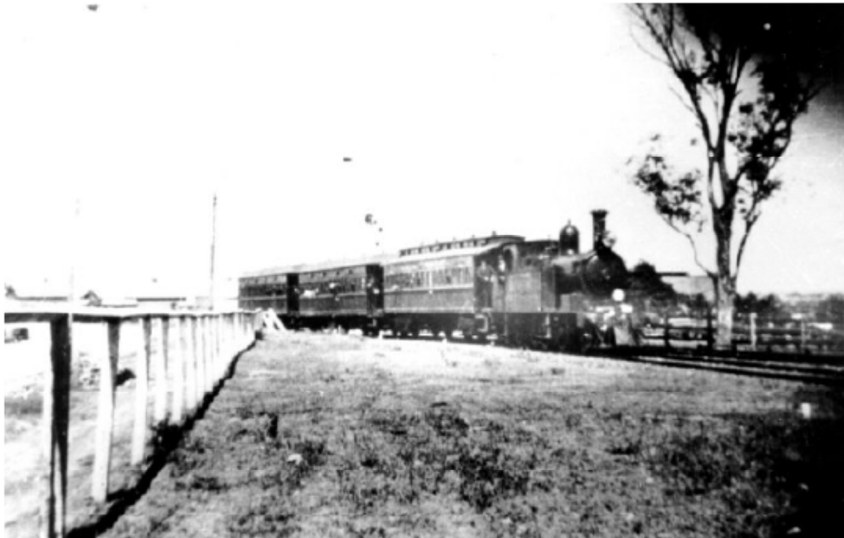
Photograph 2.4 Train entering Castle Hill goods yard and station area on opening day 28 January 1923 (source: Watson 2010)
