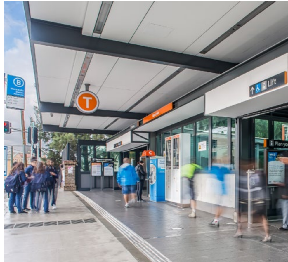
Figure 4.20 Illawarra Road station entry, upgraded in 2016
