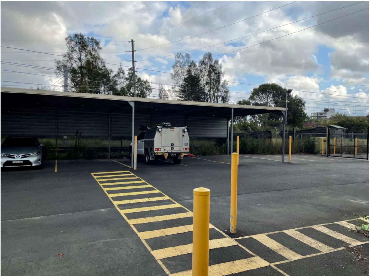
Plate 2 Image of the asphalted Belmore site office complex. Image supplied by HSEJV.
