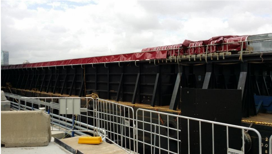
Above: Moored Barge showing steel wall for spoil containment and retractable protective cover (closed as shown)
