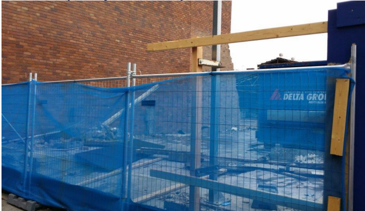
1 of 2 sections along Cope Street without hoardings.
