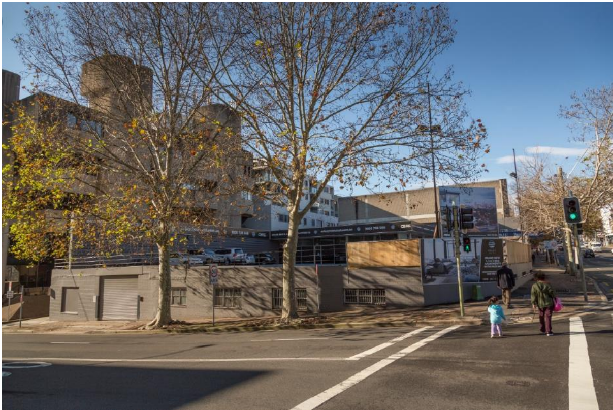
Figure 17 – Former development at Site A North
