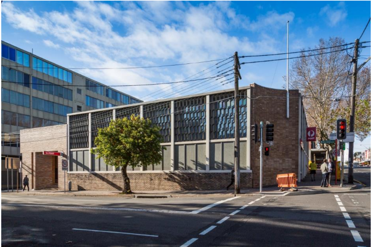
Figure 18 – Former development at Site B
