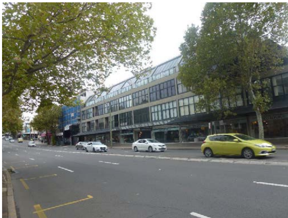
Figure 26 – Existing development to the west of the site, viewed from the eastern side of the Pacific Highway
