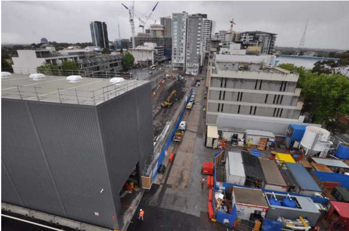
Figure 21 – Existing development of the site (October 2018)
