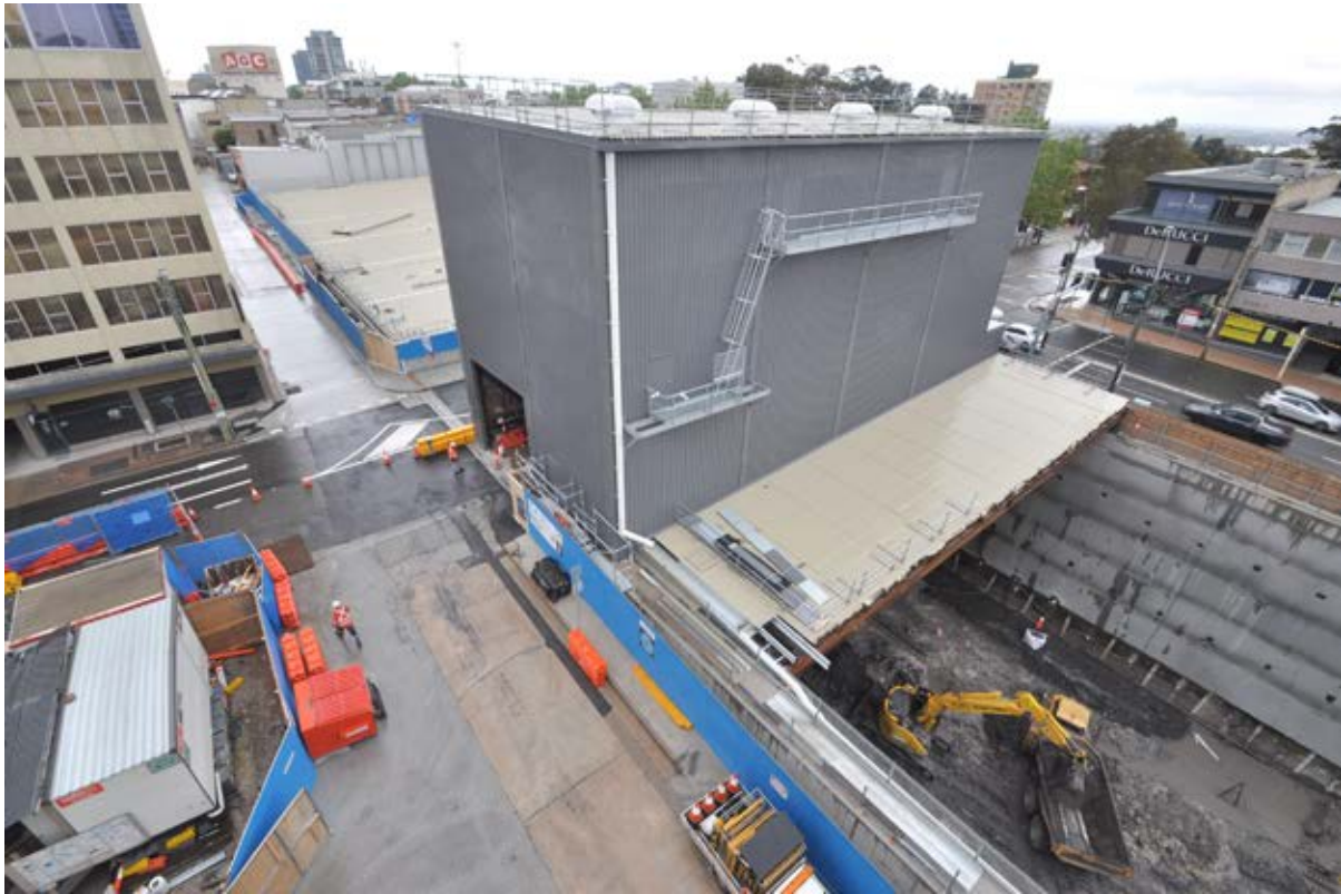
Figure 20 – Existing development of the site (October 2018)
