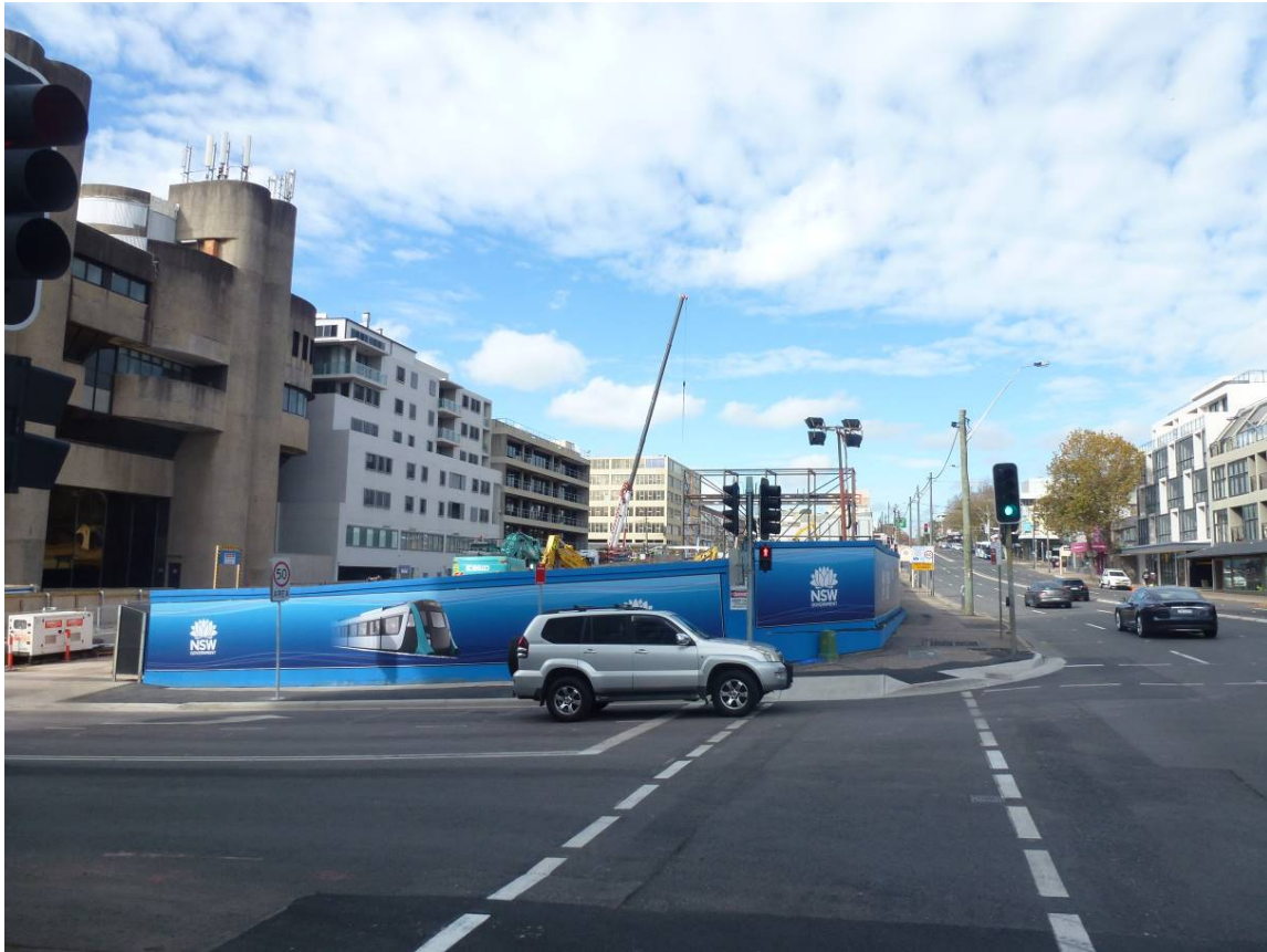
Figure 7 – Status of CSSI works on Site A as of early June 2018
