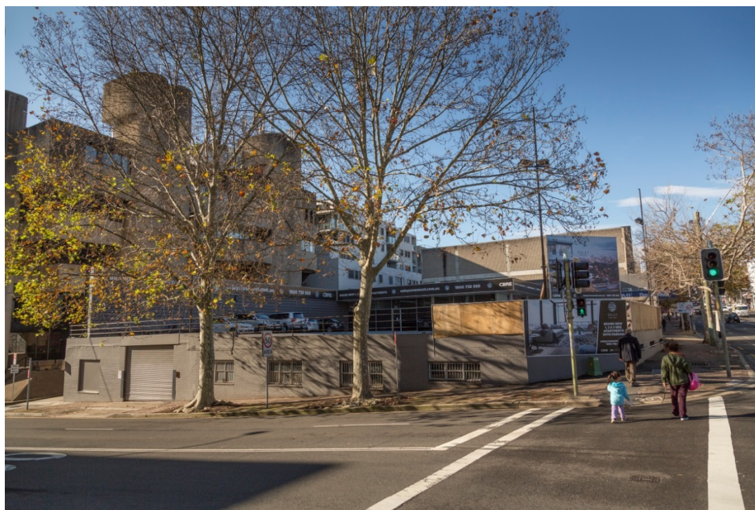
Figure 4 – Development on Site A prior to demolition works commencing
