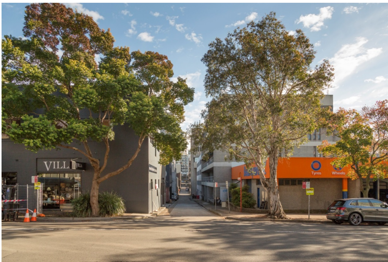
Figure 6 – Development on Site C (right) prior to demolition works commencing
