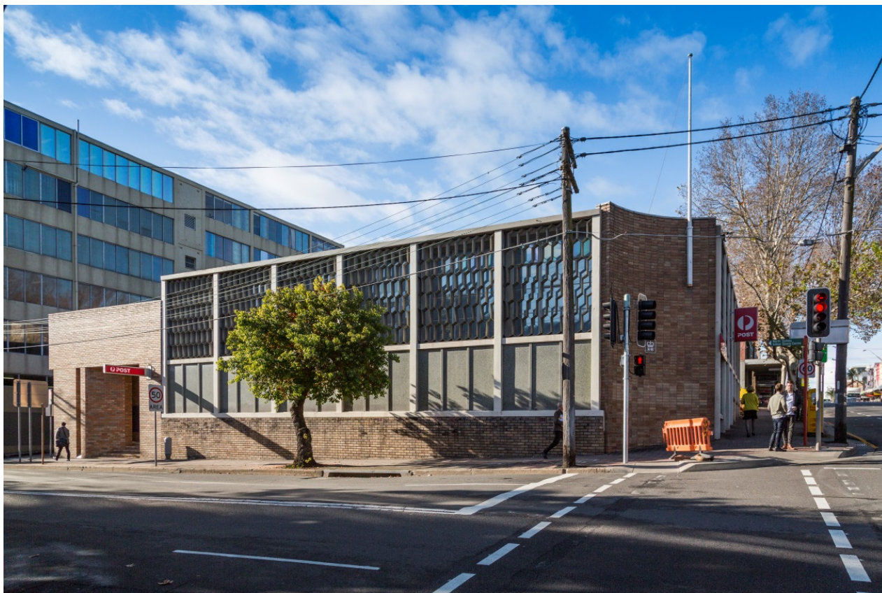
Figure 5 – Development on Site B prior to demolition works commencing
