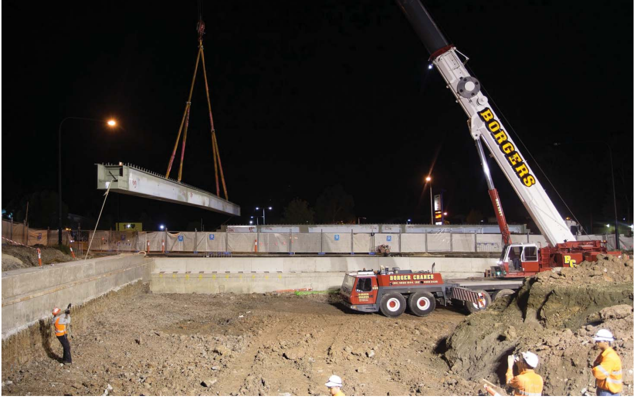
Figure 9 - Sydney Monorail Beams being re-used at the Norwest Station Site
