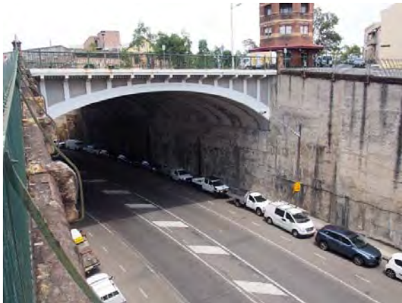
Visual separation created by sandstone cuttings along Hickson Road, and view to historic arched Bridge at Argyle Place
