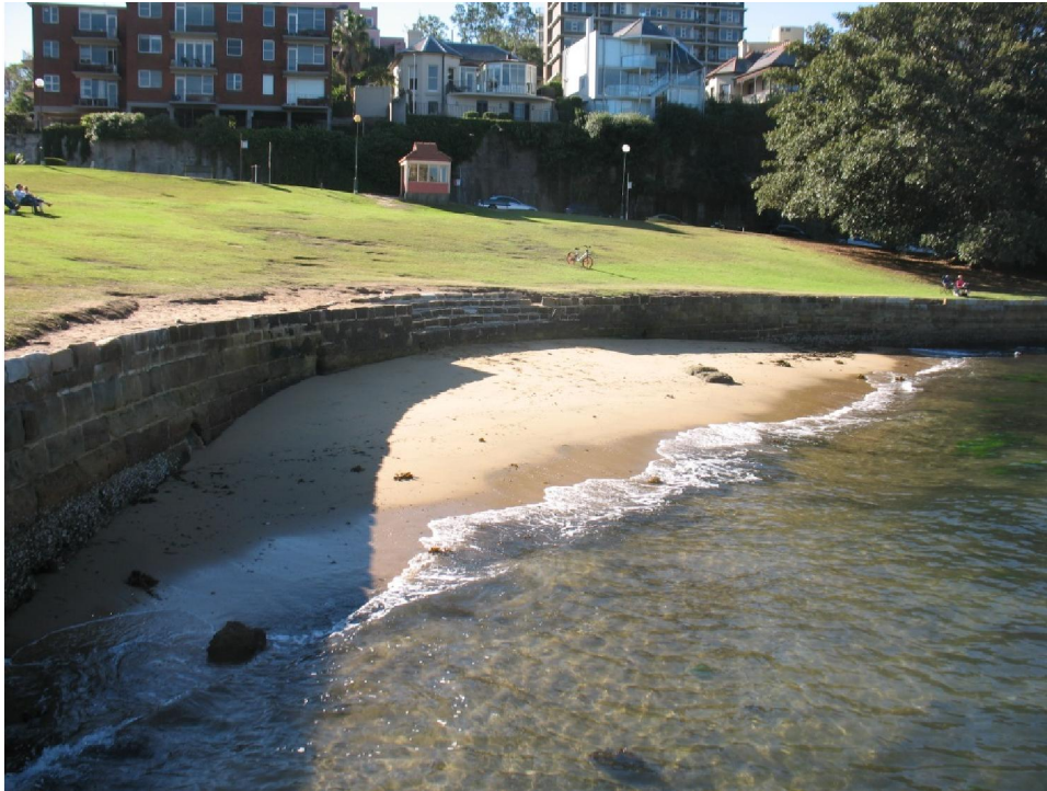
Figure 3.7. Seawall extending along the foreshore
