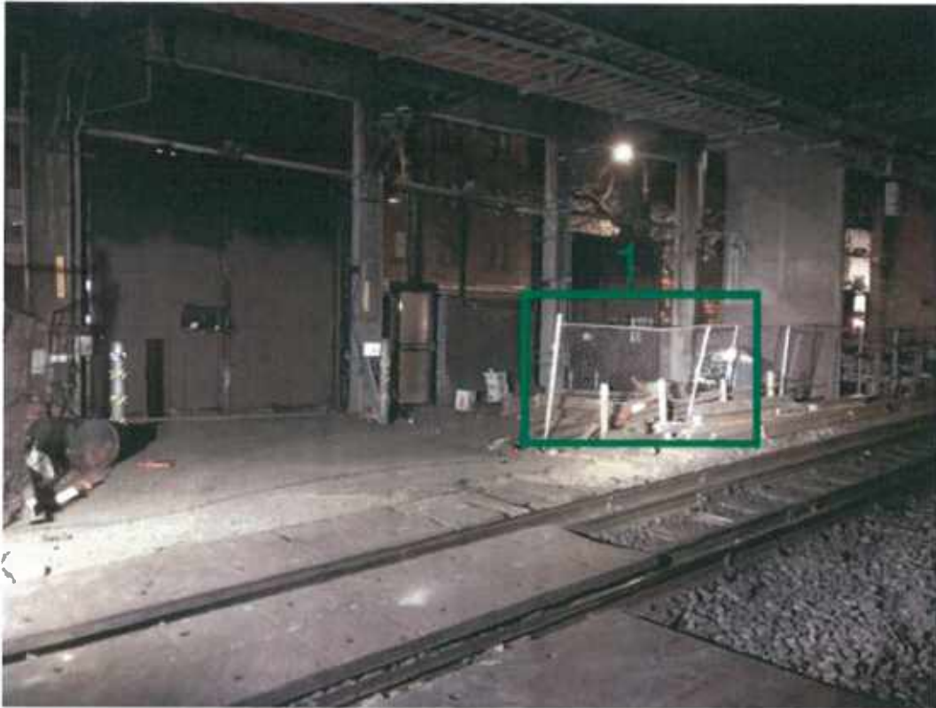
Plate 4: Area to be cleaned and used as temporary lay down.
