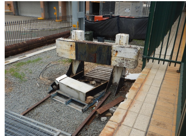
FIGURE 2.15: HARDWOOD BUFFER STOP AT THE TERMINATING END OF THE SIDINGS, ADJACENT TO PLATFORM 1, WITH REMNANT BOUNDARY FENCE IN THE BACKGROUND.
