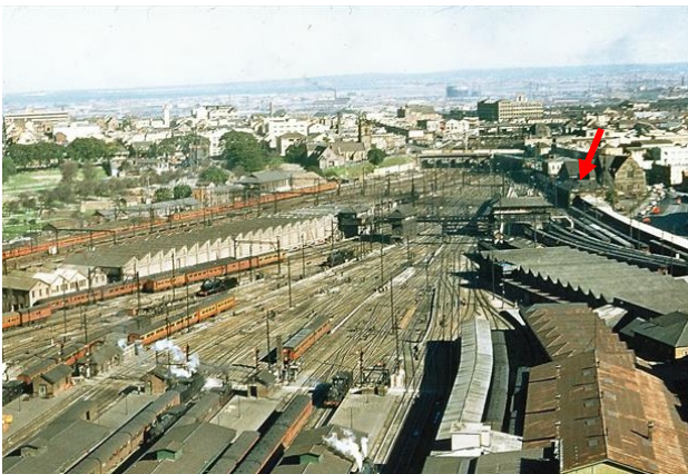
FIGURE 2.34: THIS IMAGE, CAPTURED IN THE EARLY 1950S, SHOWS MAST STRUCTURES LIKELY INSTALLED C.1934, PRIOR TO FULL ELECTRIFICATION OF PLATFORMS 1-10. MORTUARY STATION IS IDENTIFIED BY RED ARROW.
