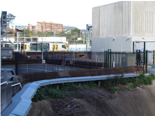
FIGURE 2.13: WESTERN BOUNDARY FENCE WHERE IT EXTENDS AROUND THE CUTTING FOR THE DARLING HARBOUR GOODS LINE.
