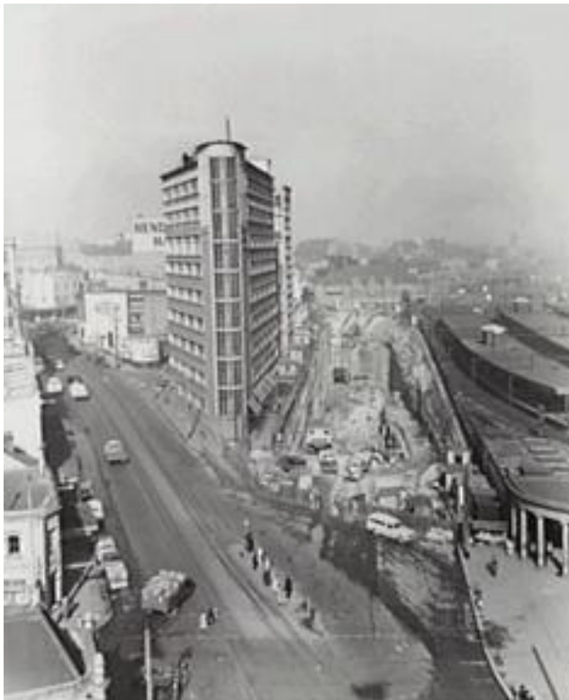
Figure 14: Photograph showing excavation of the ESR, extending across the total width of Chalmers Street. Source: City of Sydney Archives late 1940s excavation Syd Ref Coll SRC136
