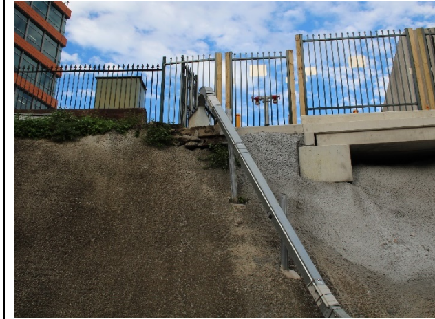
FIGURE 2.29: VIEW SHOWING JUNCTION OF EARLY STEEL PALISADE FENCE AND MODERN PALISADE FENCE AT THE NORTH END OF THE DHGL. THE TRANSITION METHODOLOGY WILL NOT AFFECT THE HERITAGE FENCE OR BRICK EMBANKMENT WALL AT THIS END.
