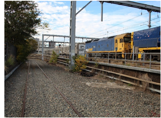
FIGURE 2.21: VIEW SHOWING MODERN FENCING INSTALLED ON THE EASTERN EMBANKMENT WALL.
