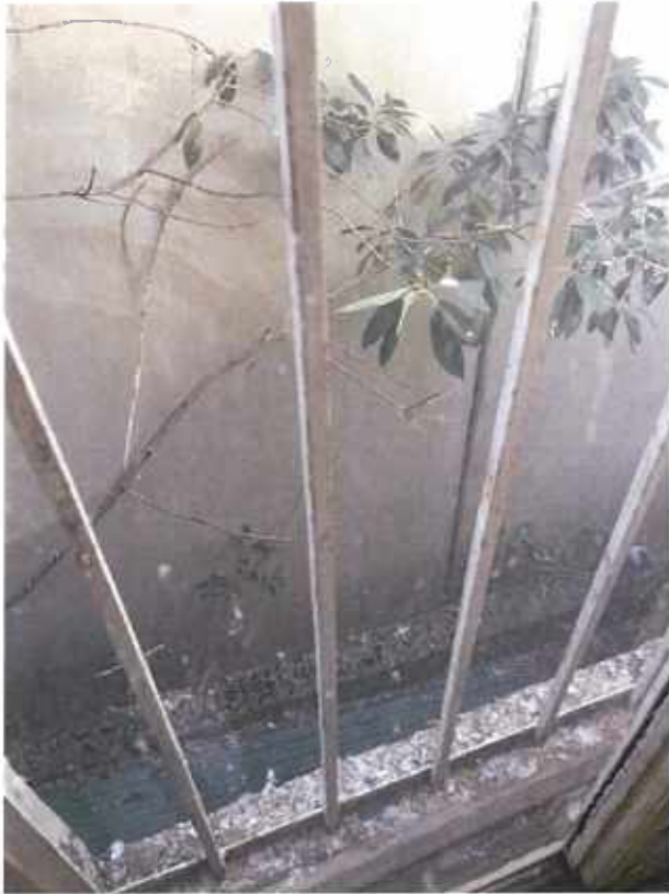
Photo of annex male toilet roof and back brick wall below
