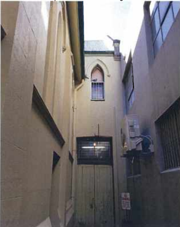
Photo of annex exterior and south corridor
