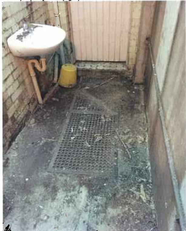
Photo of male toilet concrete floor
