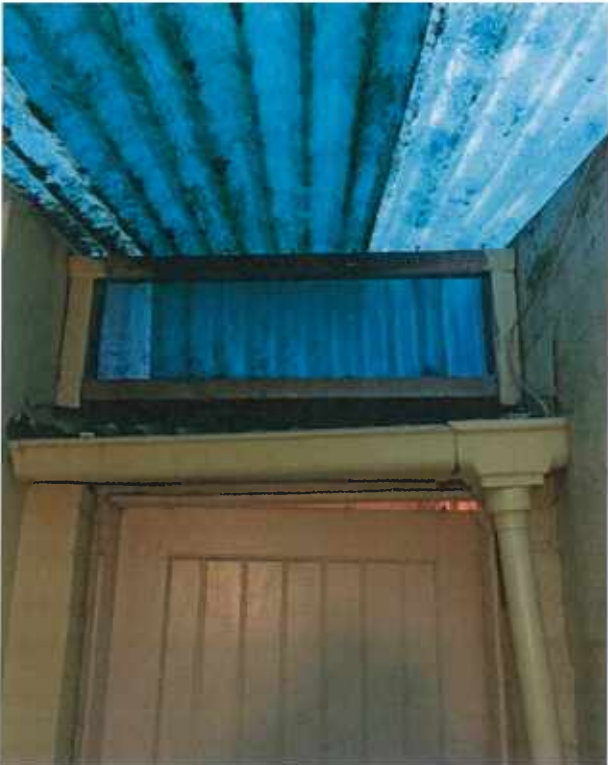
Photo of female toilet roof and door to WC (looking north)
