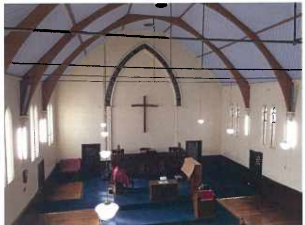
Photo of chapel interiors looking east
