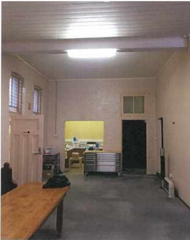
Photo of annex and kitchen (looking south). The existing kitchenette in the background
