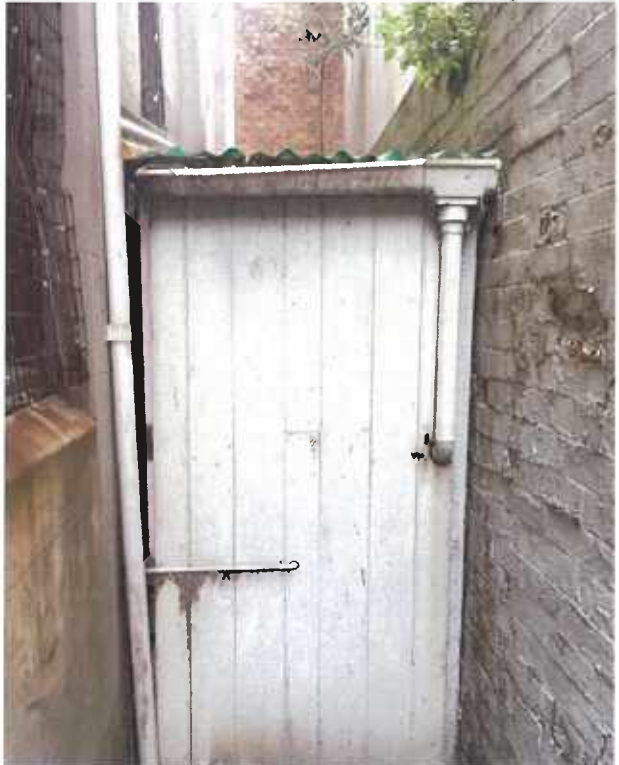
Photo of female toilet south facing timber panel wall
