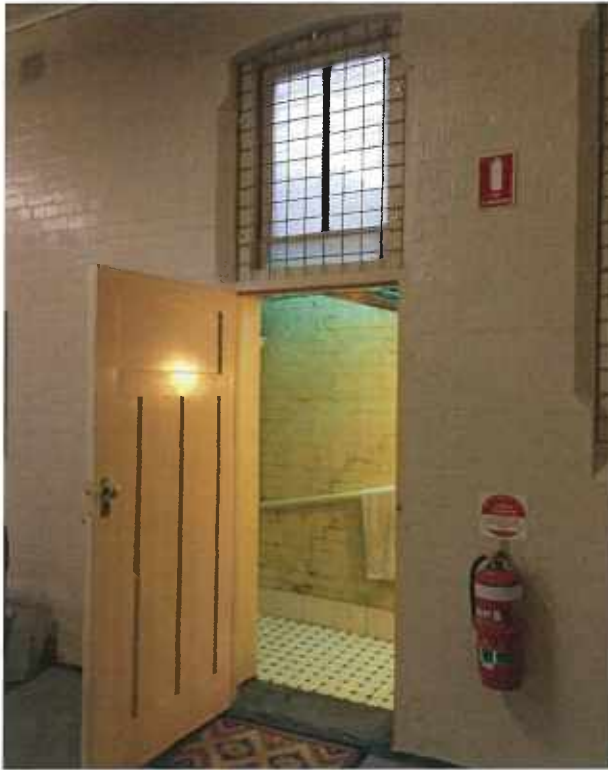
Photo of door to female toilet in the annex east wall
