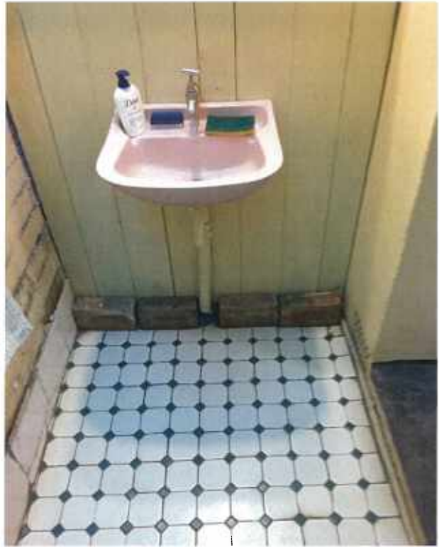
Photo of female toilet tiled floor and south timber panel wall
