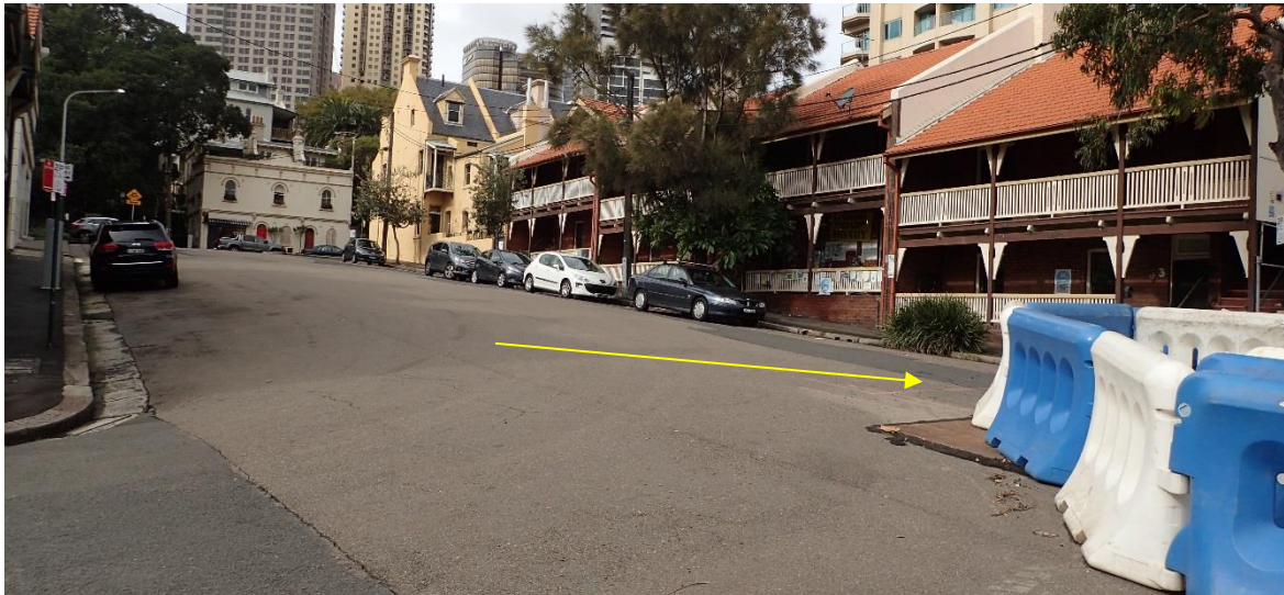
Figure 4.22 The trench along the south side of the east-west High Street return.
