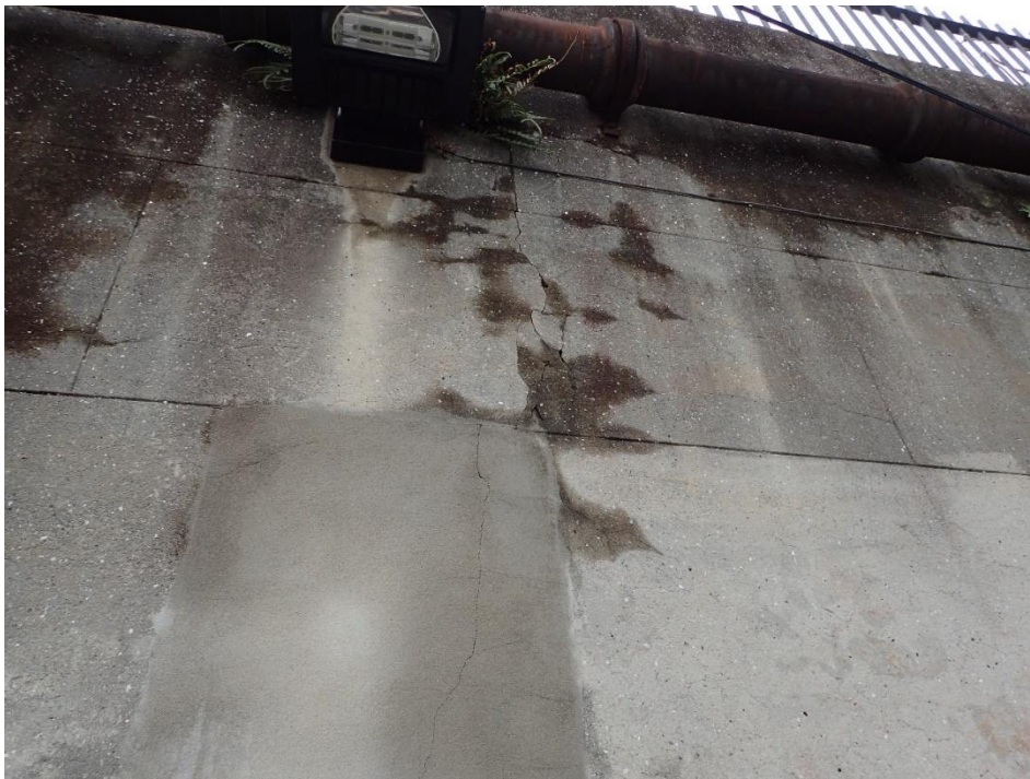
Figure 4.14 A patch of modern cement render surrounded by the original render. The white flecks are shell fragments.
