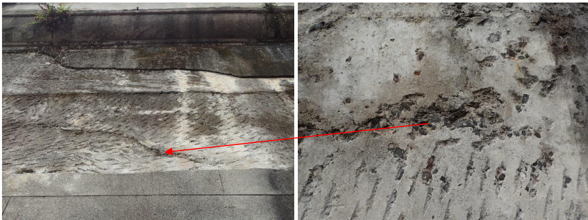
Figure 4.16 There are sections of concrete with dense gravel aggregate.
