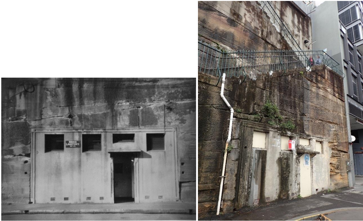
Figure 4.10 There has been little external change to the Men's Lavatory since 1934, when the photo. Left, was taken other than removal of the identifying sign ( http://www.photosau.com.au/cos/scripts/home.asp#NSCA CRS 538/049 ).
