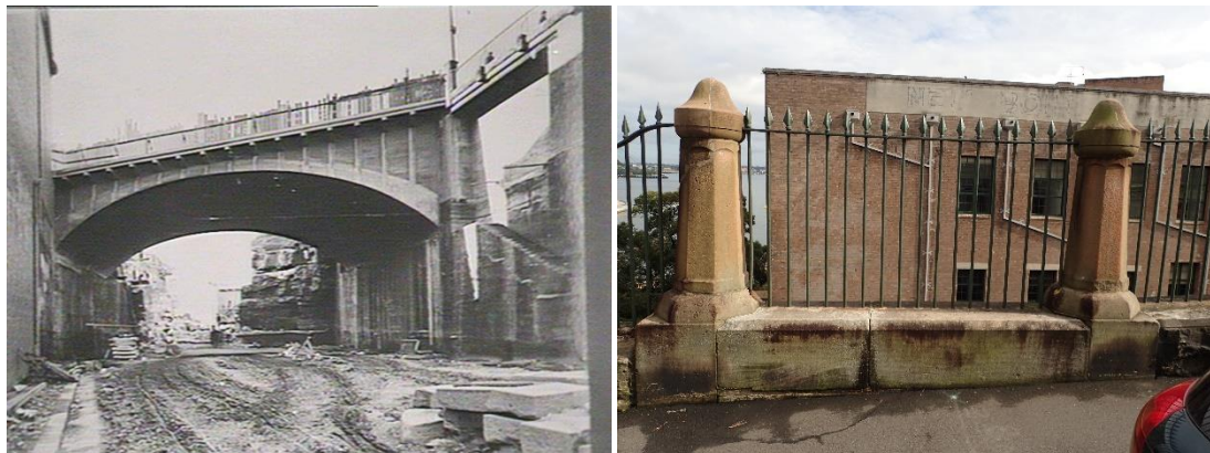
Figure 4.7 The steps do not extend to High Street in this image of the Reinforced concrete bridge, Munn St over Hickson Rd, Millers Pt. Note sandstone blocks for the construction of the wall in the foreground (left slnsw #FL1866347). It seems likely that the sandstone posts mark the access to the steps, seen here with the Dalgety Bond Stores beyond.
