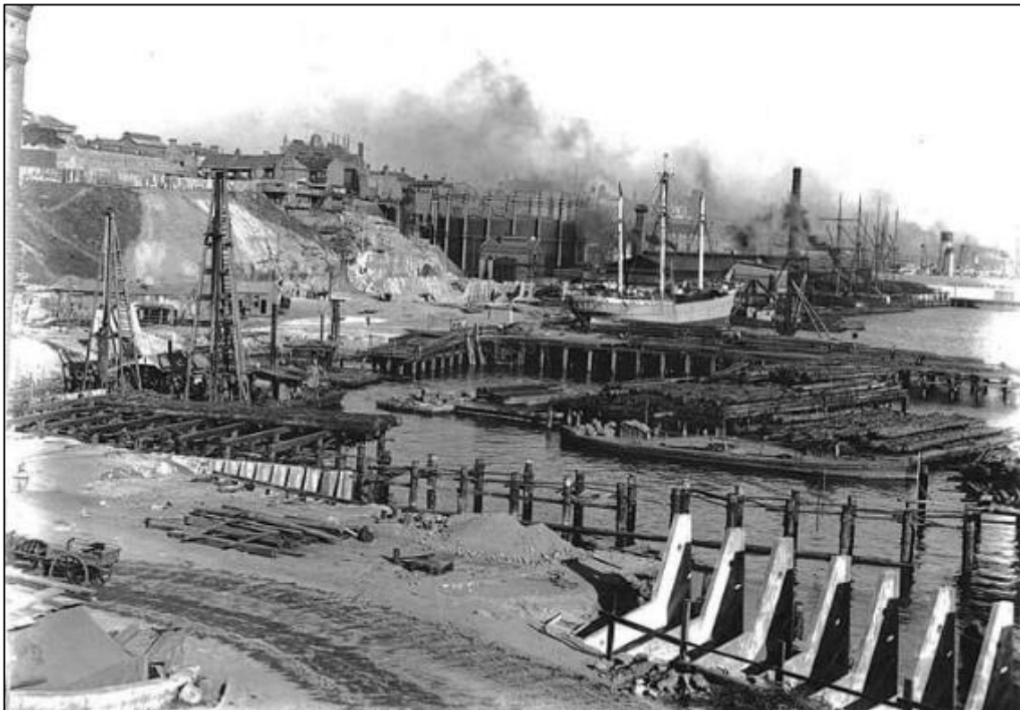
Figure 2.10 Photograph taken 1909 of the reconstruction of the East Darling Harbour wharves to the north of the Gas Works. Note that the retaining wall supporting High Street has not been built (View of the reconstruction of Darling Harbour from Millers Point showing Dalgetys Wharf No.1 partly completed. The sailing ship 'Macquarie' is shown being unrigged before being reborn as the coal hulk 'Fortuna' Dated: 1/1/1909 Digital ID: 9856_a017_A017000007. https://www.records.nsw.gov.au/series/9856?title=&page=5 ).
