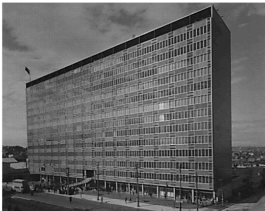
Figure 1 MLC Building North Sydney 1957. Note the open north elevation, the construction of which is similar to the south elevation.
