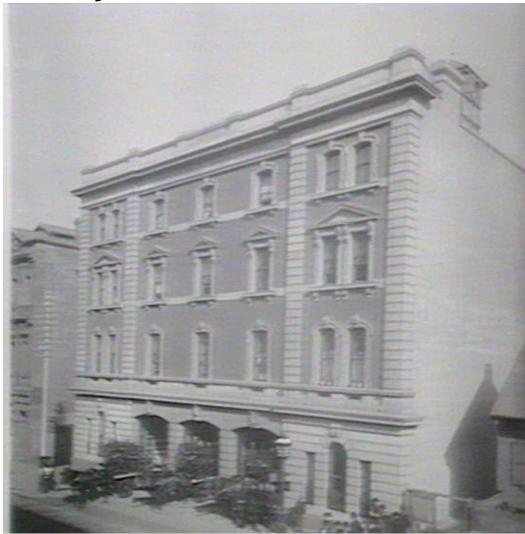
Figure 4 Fire Station no 1 c 1900 . The building is constructed from face brick with rendered detail.
