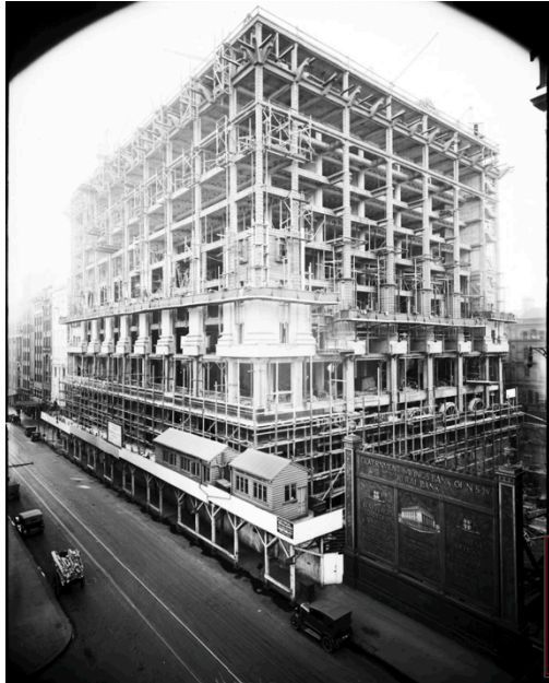
Figure 1 48 Martin Place under construction c1926 looking north along Pitt St. Note the concrete encased framing which on the principal facades are to be terracotta clad. Note also the relatively lower northern building on Pitt St, the upper parts of the north wall of the building were designed to be exposed.
