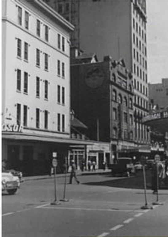
Figure 3 Masonic Club, south elevation c 1960 . Note the relatively lower scale and earlier building to the south. It would be expected the rendered masonry shown in the image survives and beneath the present 4 th floor the south wall will be unfinished common brick work.
