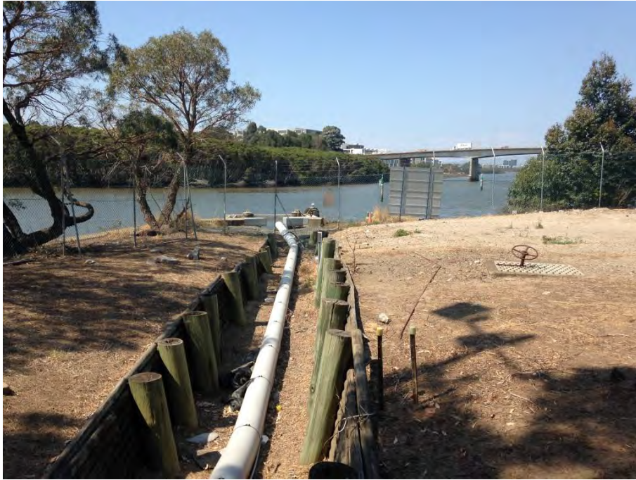
Plate 4.2: Hardstand area and Gore Bay pipeline adjacent to the wharf.
