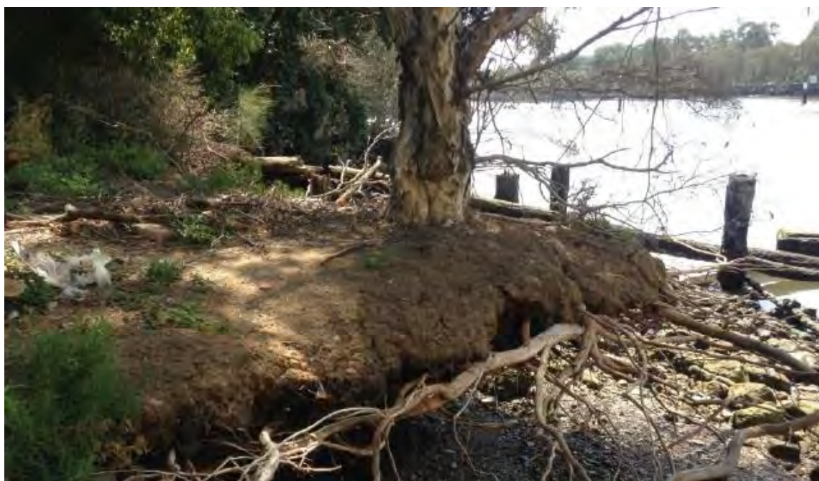
Figure 3.5 Recent photograph of timber piles at the Shell Refineries Jetties location
