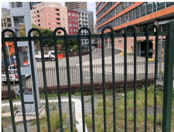
Figure 7: The sandstone and iron fence from Platform 0/1 (Source: Sydney Metro, 2018).
