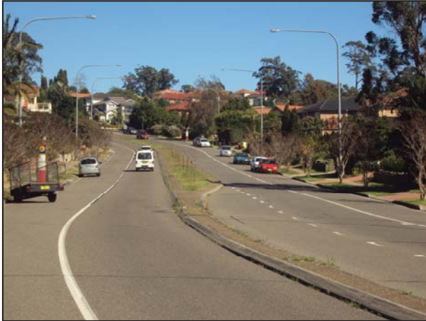
Figure 2-6: County Drive looking south towards Castle Hill Road
