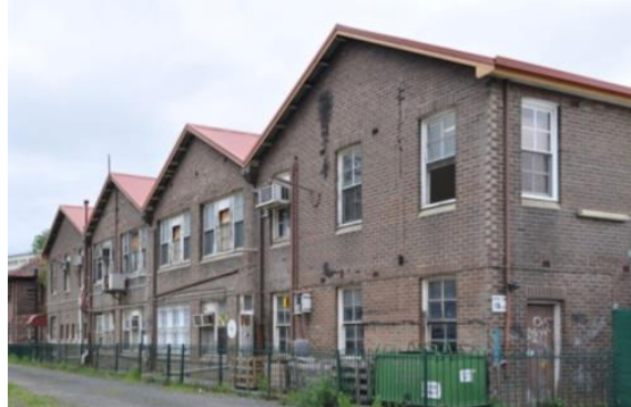
Figure 10: The Cleaners Amenities building (Source: Rappoport, 2013).
