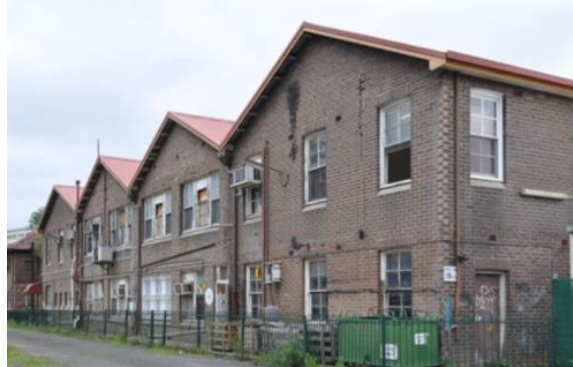
Figure 10: The Cleaners Amenities building (Source: Rappoport, 2013).
