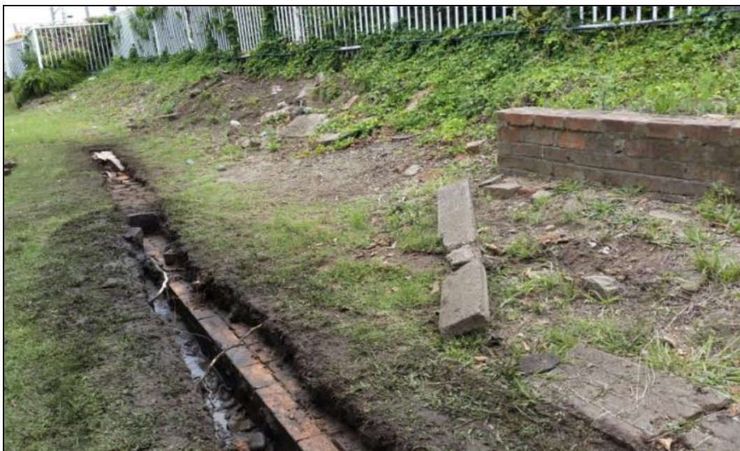
Photo 5 - Platform structure at Hamilton Railway Station classified as a 'work' by the project archaeologist - Wickham Transport Interchange project, 2015
