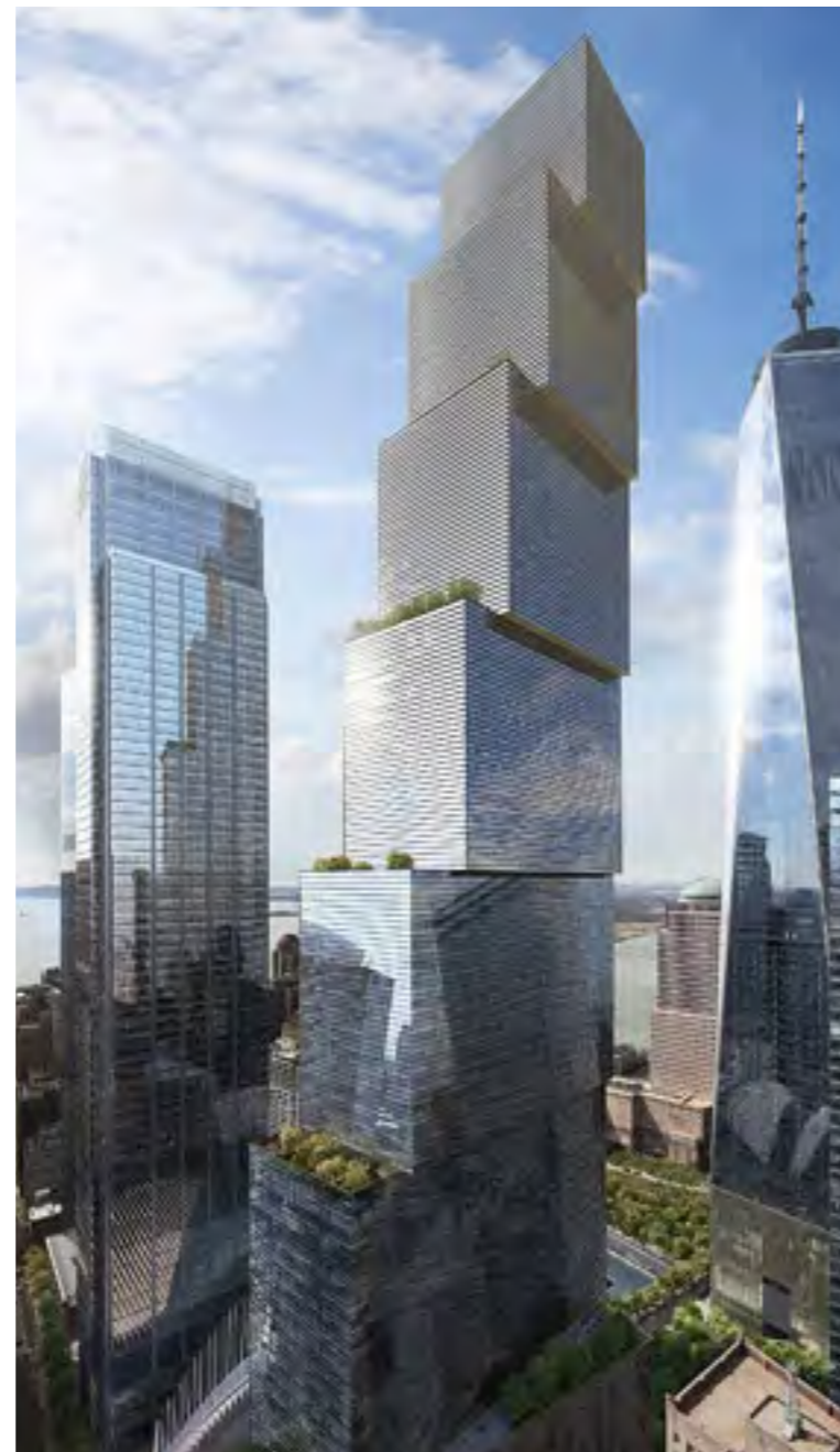
2 WORLD TRADE CENTRE / BIG / UNDER CONSTRUCTION
