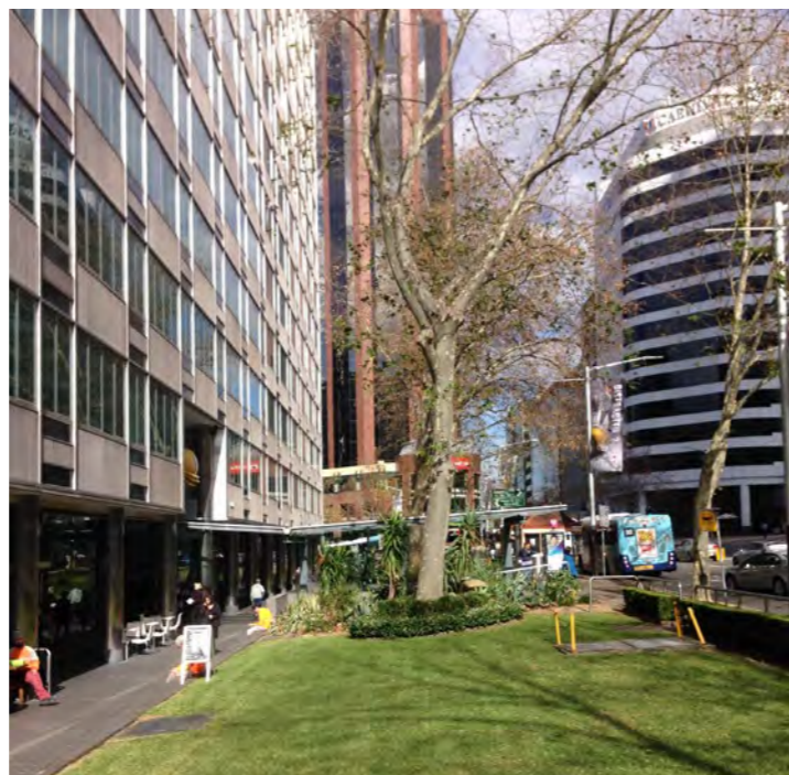
MILLER STREET SPECIAL AREA IN FRONT OF MLC BUILDING
