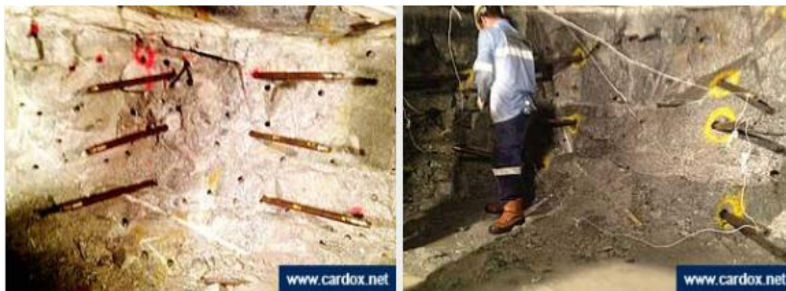
Figure 4: Use of Cardox to remove tunnel rock (source: http://www.cardox.net )
