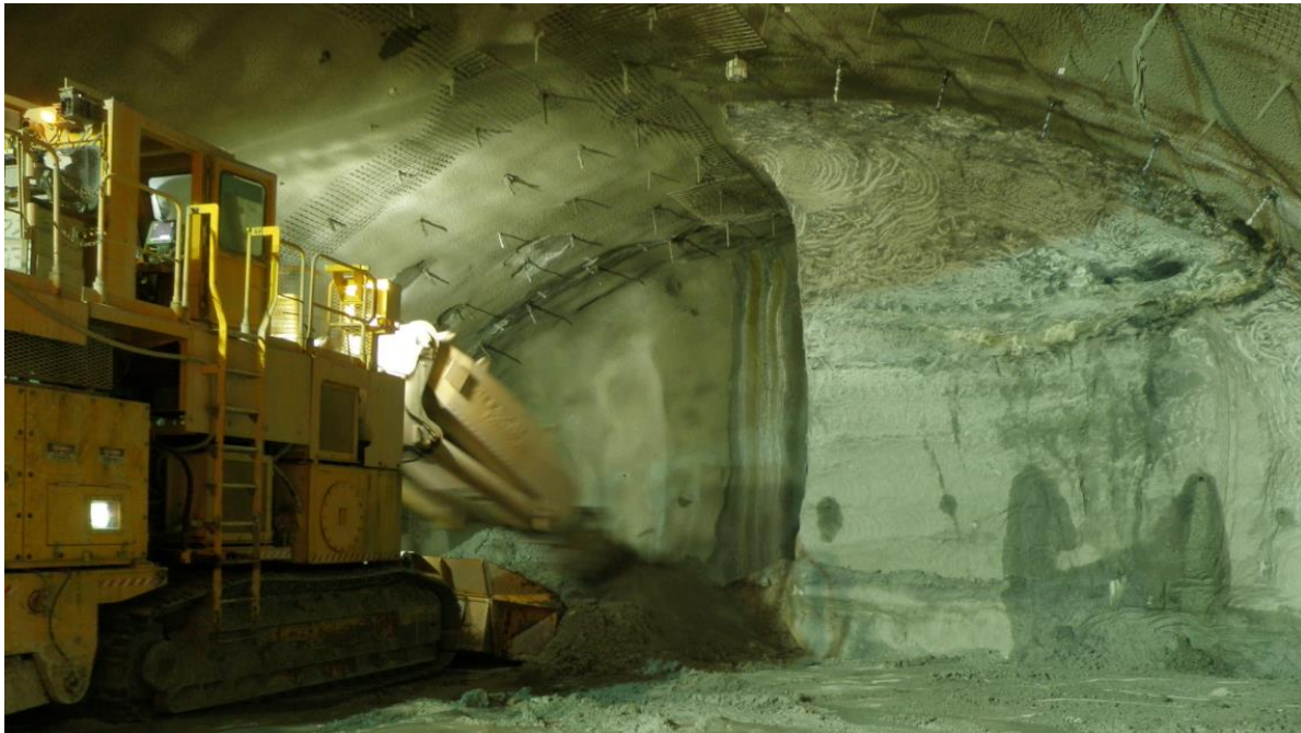
Figure 3: A roadheader excavating an underground cavern (Airport Link, Brisbane)
