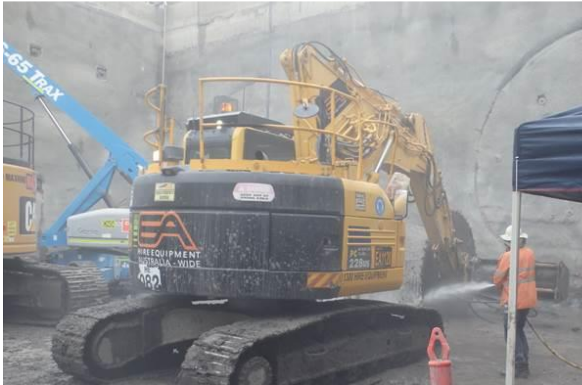
Figure 5: Use of an excavator mounted rock saw (single blade)
