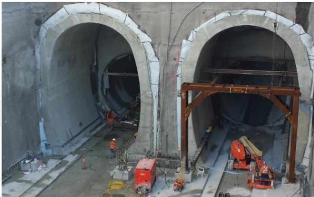
Figure 8: Nozzle and stub tunnel – prior to TBM re-launch
