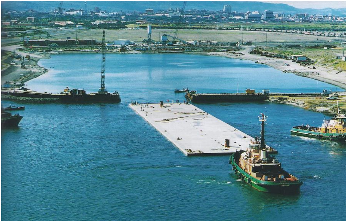
Figure 6: – A tunnel segment being towed out of the Port Kembla casting basin (source: National Geographic, photographer: Margaret Rush)
