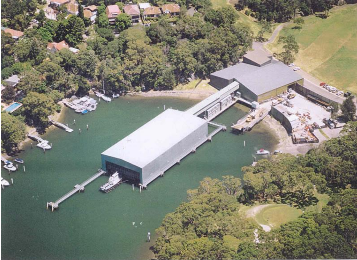
Figure 10 – North Side Storage Tunnel Barge Loading Shed at Tunks Park
