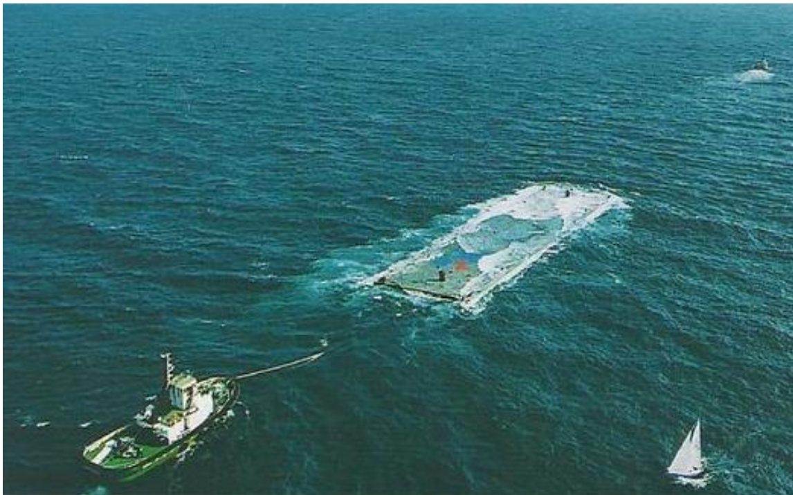
Figure 7: – tug towing the first segment from Port Kembla to Sydney Harbour (source: National Geographic, photographer: Margaret Rush)
