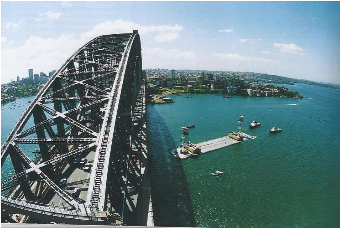
Figure 8: – Tugs manoeuvre the fourth section into position for sinking (source: National Geographic, photographer: Margaret Rush)
