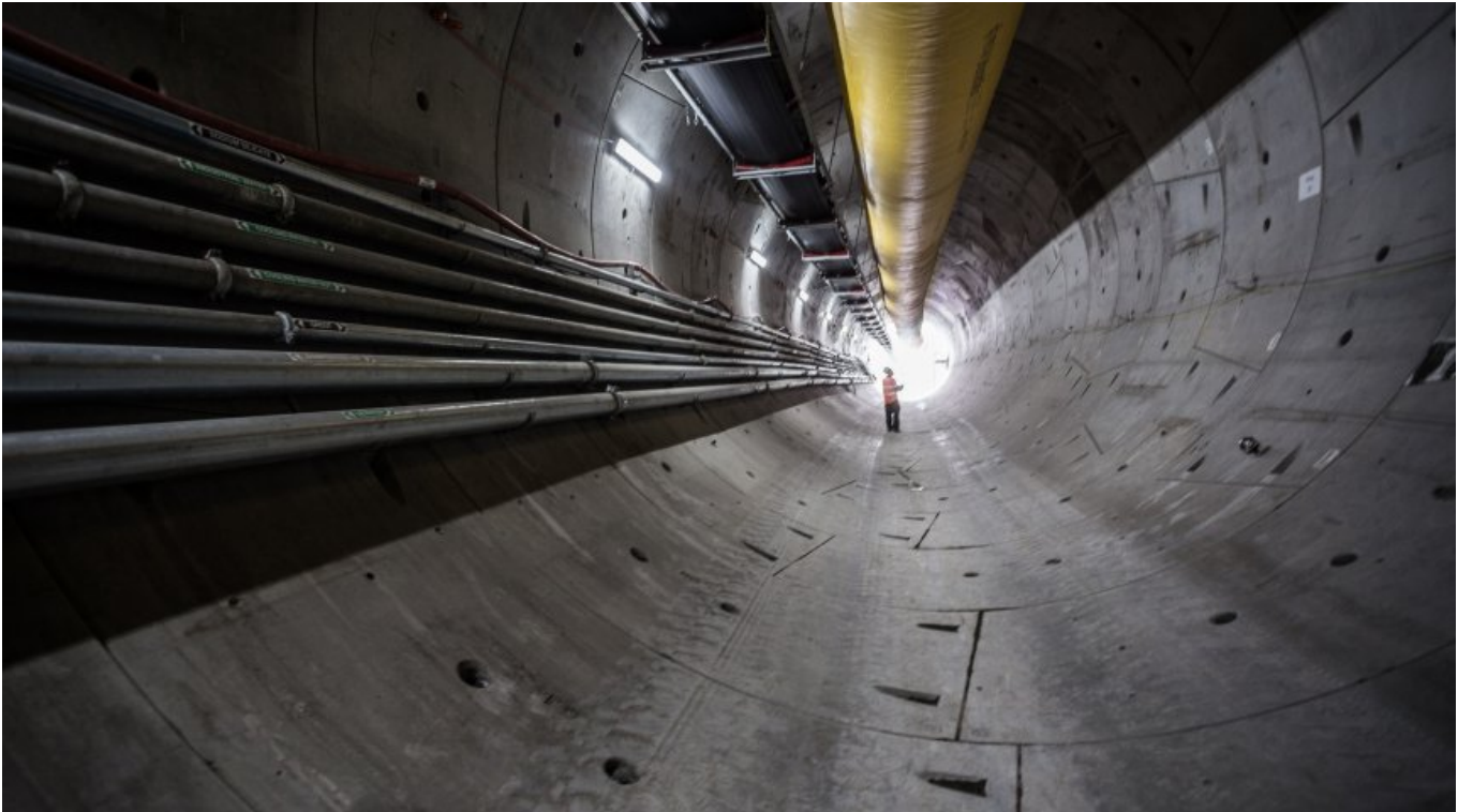
Figure 2 – Inside a Tunnel at the Bella Vista Station site
