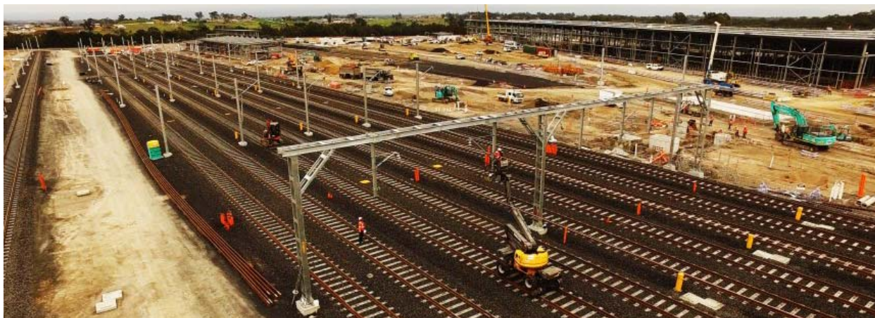
Figure 4 – Rail Tracks being laid at the SMTF Site
