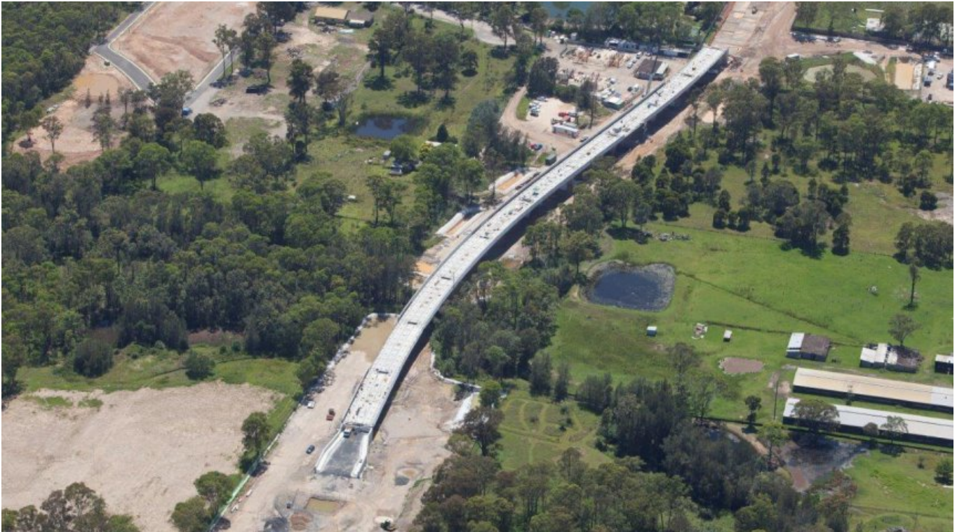
Figure 3 – Construction of the Skytrain at Second Ponds Creek
