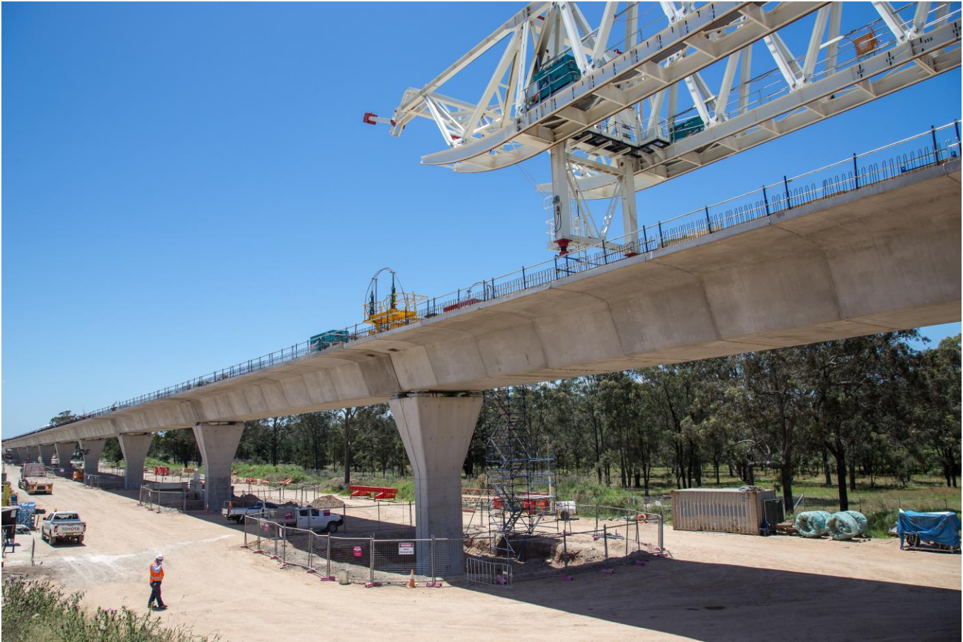
Figure 3 – Construction of the Skytrain Viaduct at the Kellyville Site
