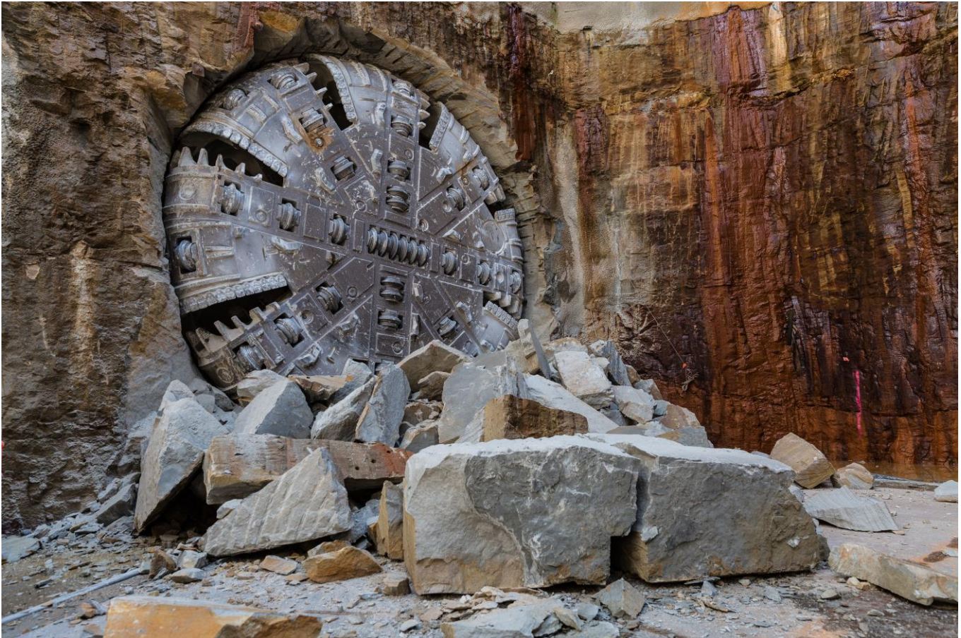
Figure 2 – Break-Through of TBM Maria at the Epping Station site on 29 October 2015
