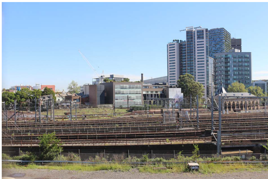
EXISTING VIEW ACROSS RAIL CORRIDOR
