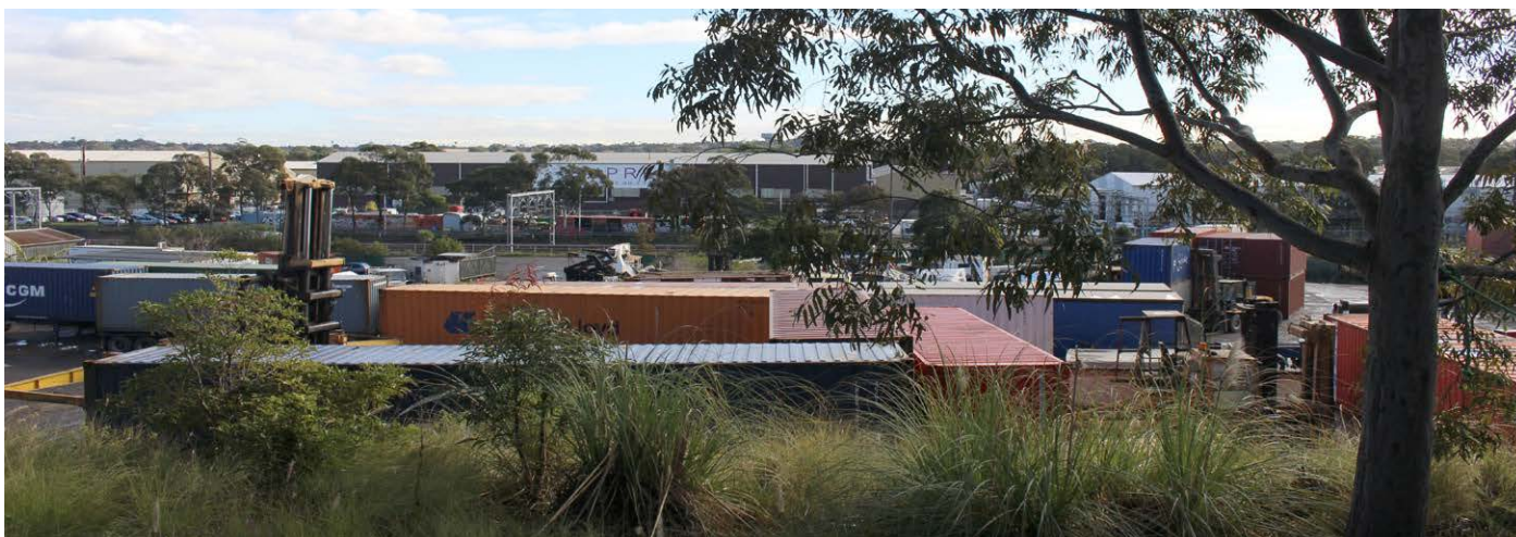
VIEW WEST OVER THE SYDNEY TRAINS NETWORK SYSTEM BASE
