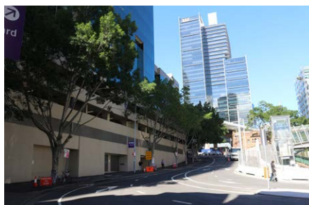
POWER UPGRADE ALIGNMENT VIEWS ALONG (L-R) HUNTER STREET, MARGARET STREET, NAPOLEON STREET
