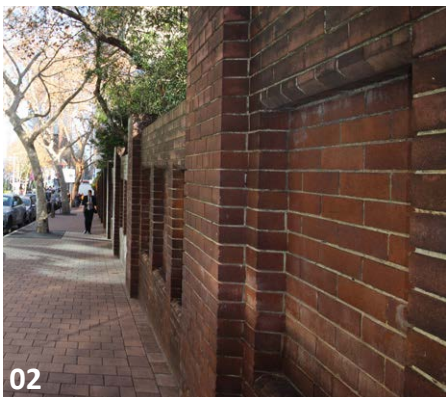
01 HERITAGE LISTED 'MONTROSE' BUILDING 02 MONTE SANT' ANGELO MERCY COLLEGE BOUNDARY WALL
