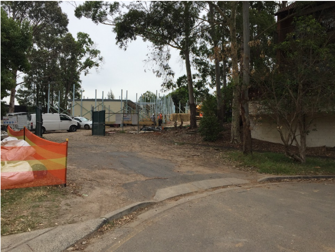
Plate 3: View northwest across the Artarmon construction site from Barton Crescent
