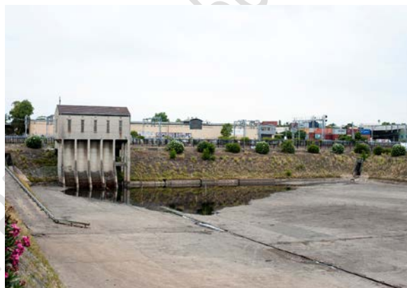
Plate 25: View south across Sydenham Drainage Pit and Pumping Station
