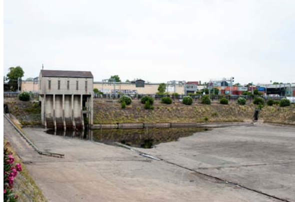
Figure 193: View south across Sydenham Drainage Pit and Pumping Station
