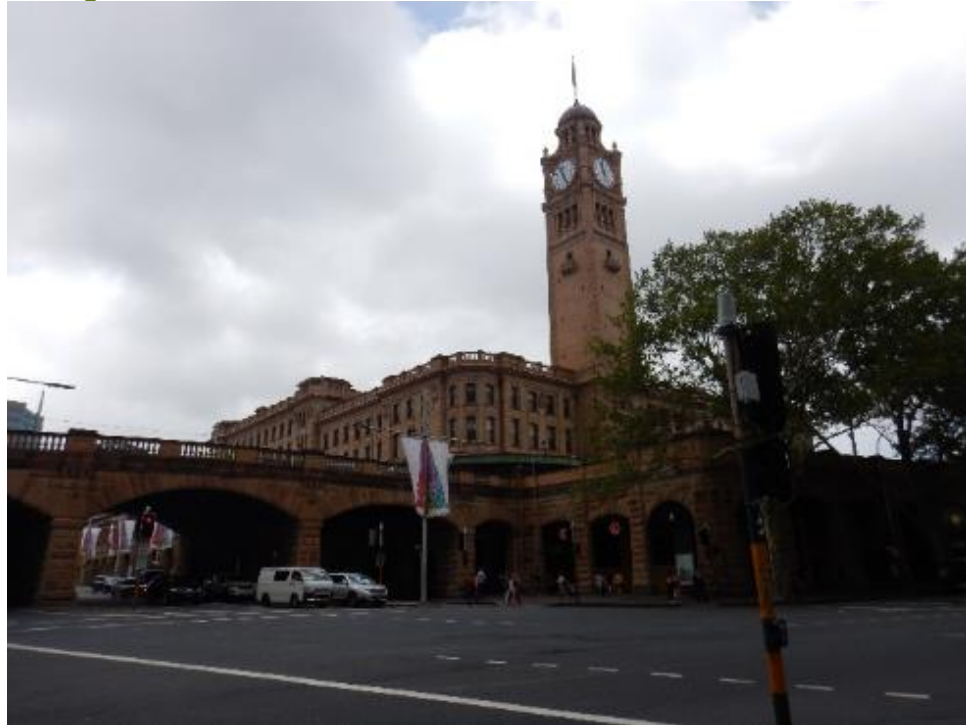
Figure 170: Sydney Terminal and Central Railway Station Group. Artefact Heritage 2015.
