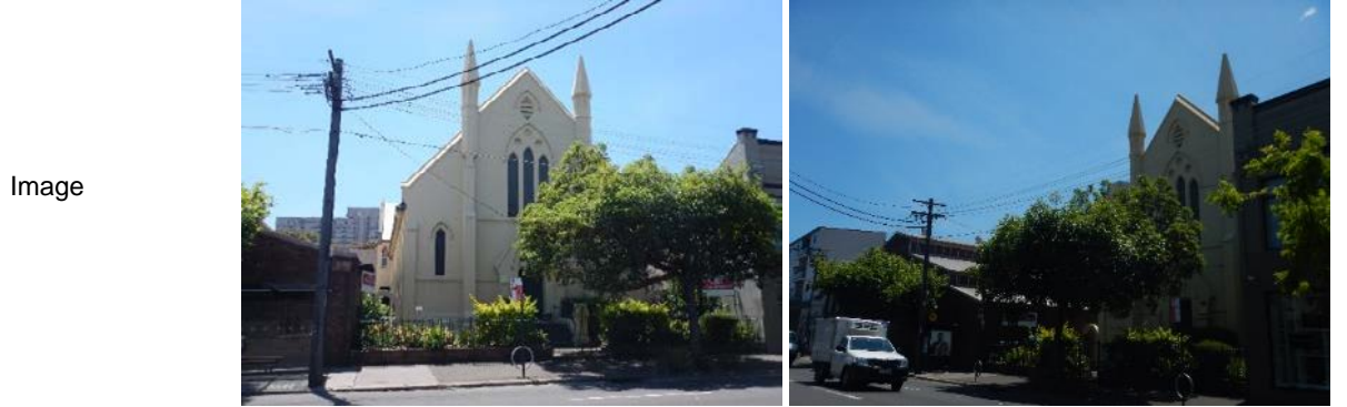
Figure 180: Congregational Church and street context. Artefact Heritage 2015.
