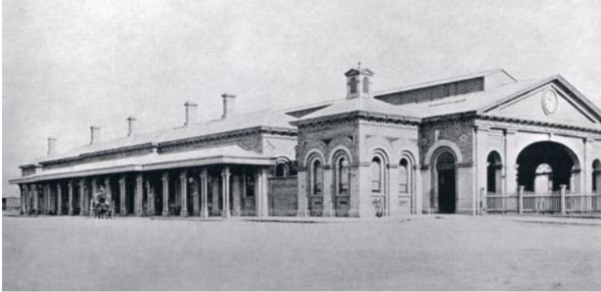
Figure 167: The Second Sydney or Redfern Station, from the west, with train shed covering two platforms. Source. McKillop.149
