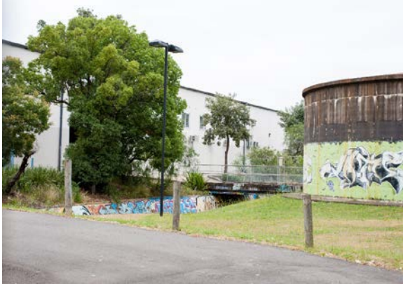
Figure 192: View southwest of Murray Street showing canal
