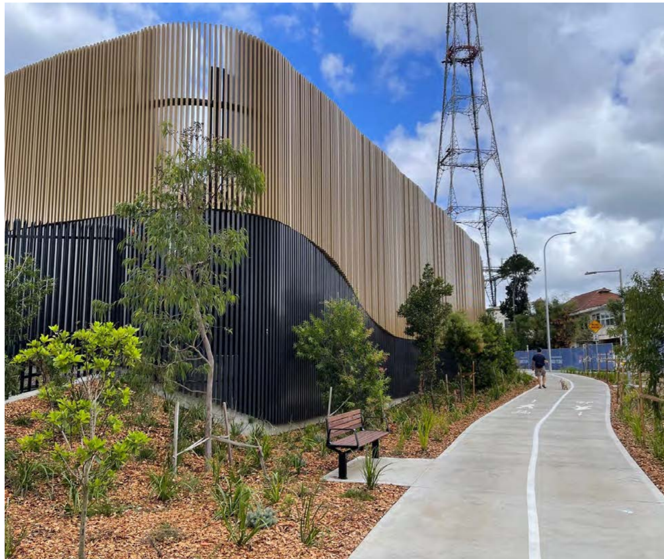
Image: Frank Channon Walk extension next to the Sydney Metro Chatswood maintenance facility.
