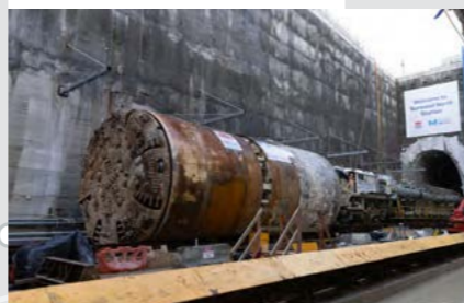
Burwood North Station
