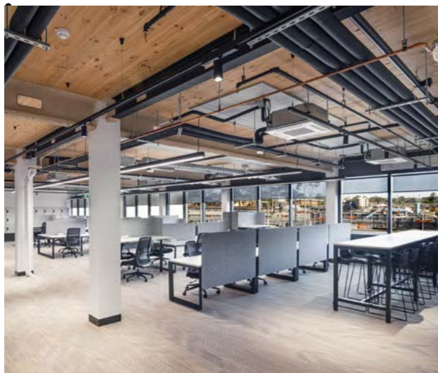
Image: Cross laminated timber used in floor panels to reduce structural steel at the St Marys Project Office.
