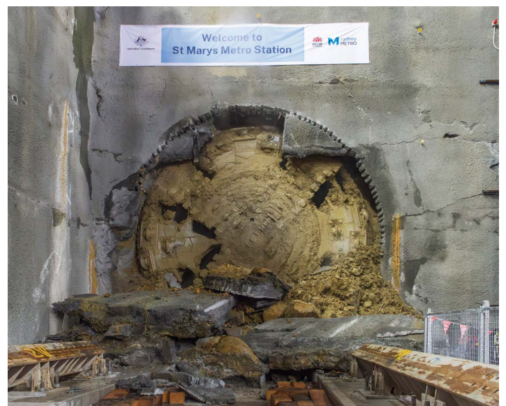
TBM Catherine was the first machine to finish tunnelling.
