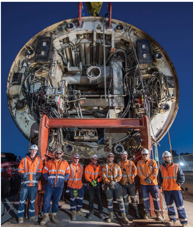
Middle shield from TBM Eileen's lifted out at Bradfield.
