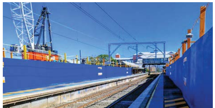
Construction hoardings on the platforms at St Marys Station.
