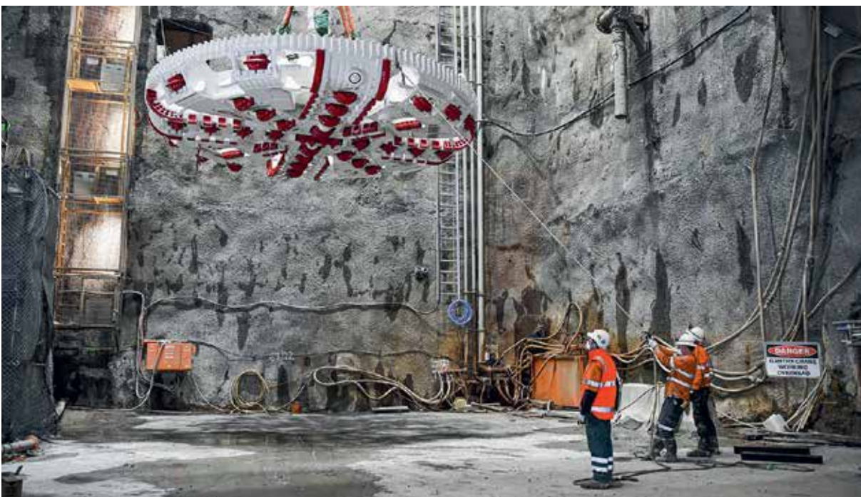
Tunnel boring machine cutter head being lowered into a shaft.
