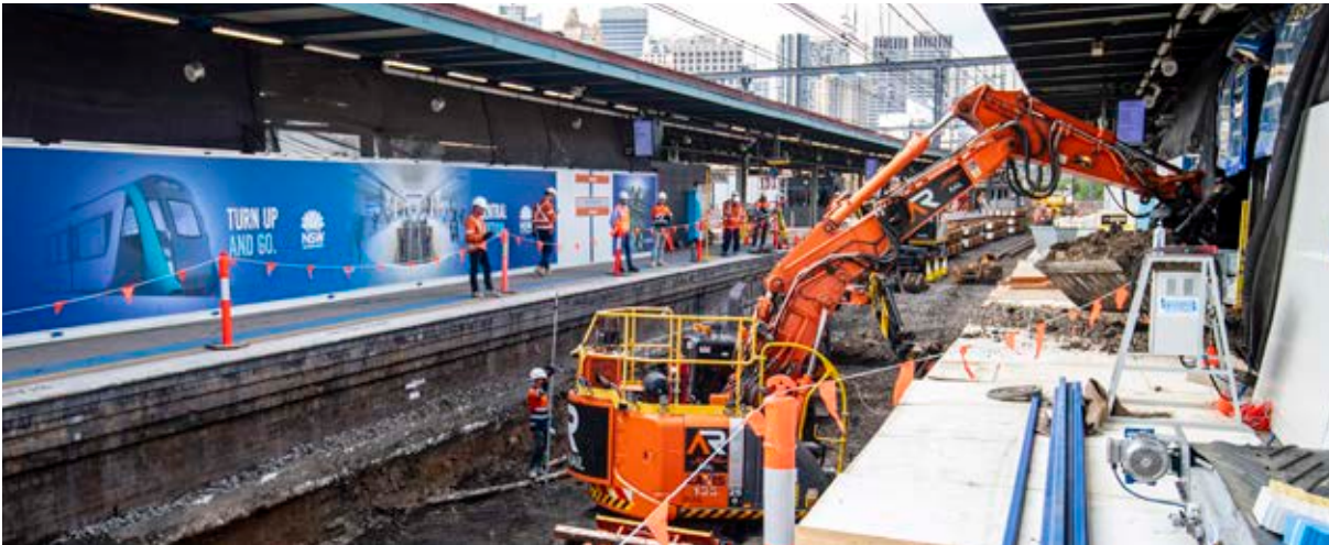
Major construction work at Central Station.
