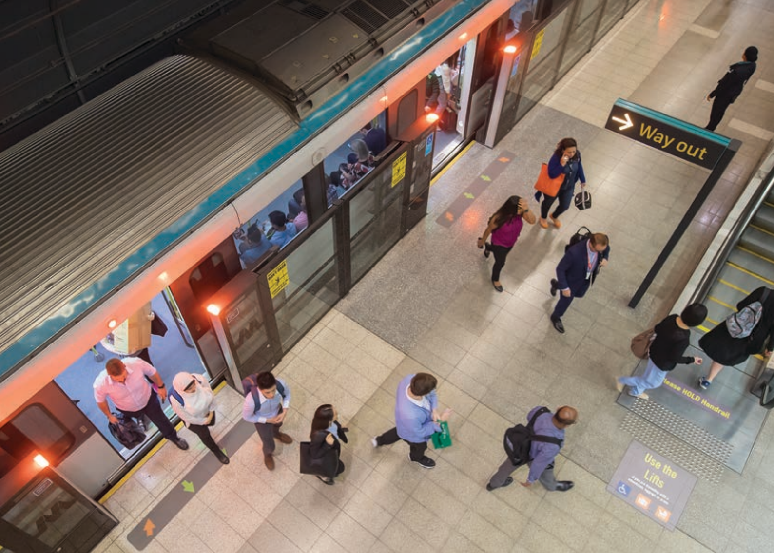
The platform screen doors allow trains to get in and out of stations faster.
